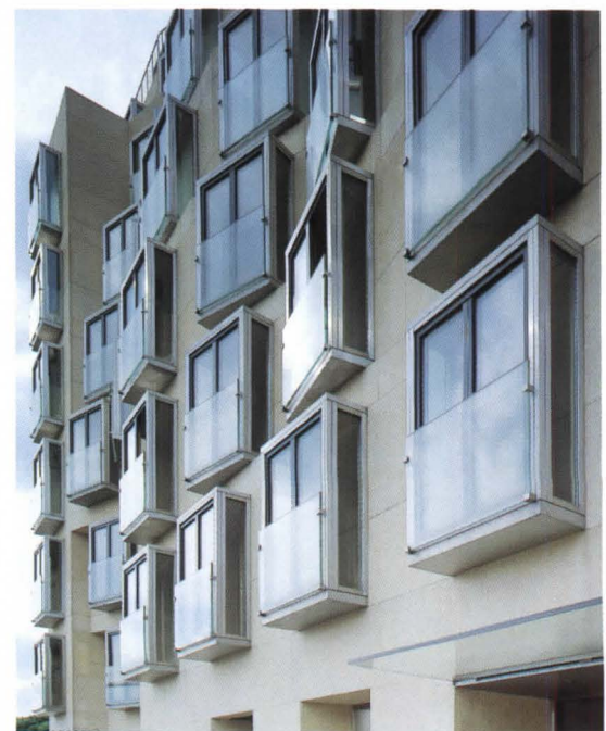
The composition of the façade facing the square (facing page, top), is comparatively conservative; in a subtle subversion of Berlin's strict design regulations, Gehry installed the window-panes on the first and fourth floors at an angle (top). The architect undulated the building's rear, south façade (facing page, bottom); and the angled projecting window frames create secondary rhythms (above).
