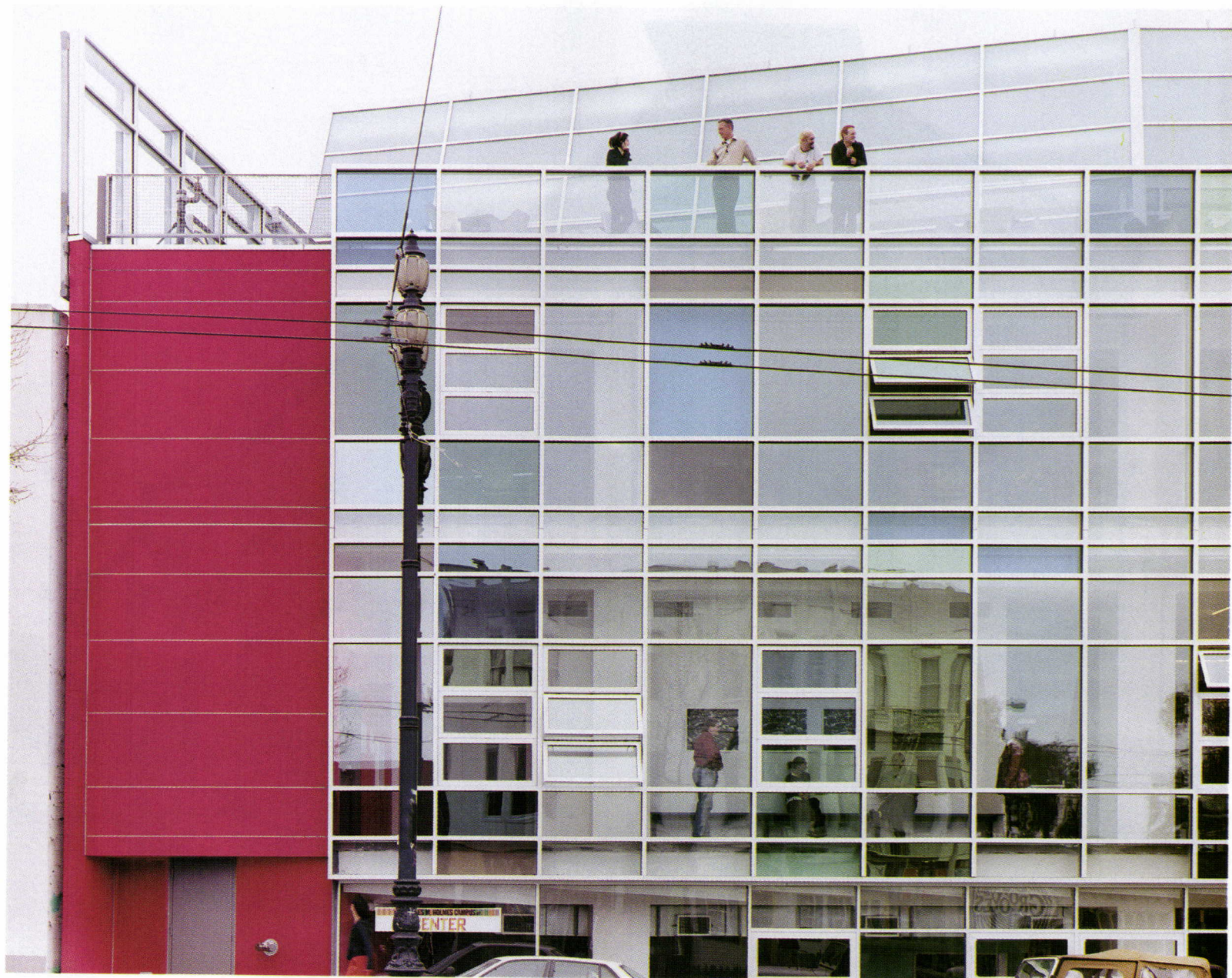
A strip of the red stucco cladding used on the center's Waller Street façade reappears on the otherwise glazed Market Street façade (above, at left). Gradiated tints of colored glass on the Market Street curtain wall play on the modernist metaphor of transparency. In a sort of peek-a-boo theme that pervades the entire building's design—the architects' conceptual and practical response to the homosexual notion of being "in" or "out" of the closet—some panes allow for more visibility into the center than others.
