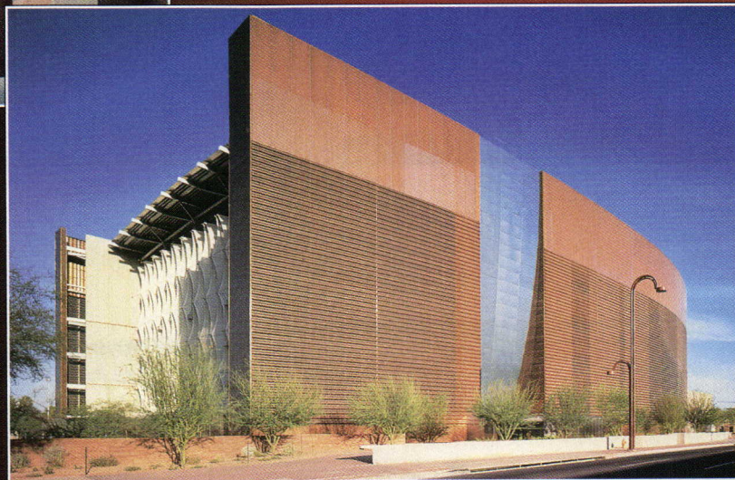
Phoenix Central Library, Phoenix, Ariz. bruderDWLarchitects
