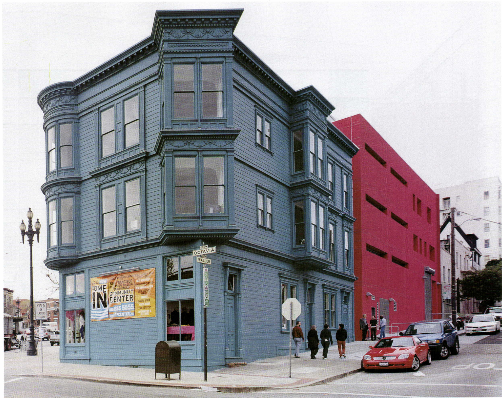
Though fiery red in color, the center's Waller Street façade is purposefully more opaque and private than the one on Market Street, so visitors have the option of making a discreet entrance. Waller Street's not always quiet, however: The loading dock was designed to double as a stage for bands during block parties. Colored lights in the atrium on Market Street signal a party inside the center (facing page, top left). The center's largest meeting space, the Rainbow Room (facing page, top right), can accommodate 350 people. The fourth-floor lounge overlooking the atrium has a view out to Market Street (facing page, bottom right). A hallway on the third floor overlooks a Baptist church on Waller Street (facing page, bottom left).
