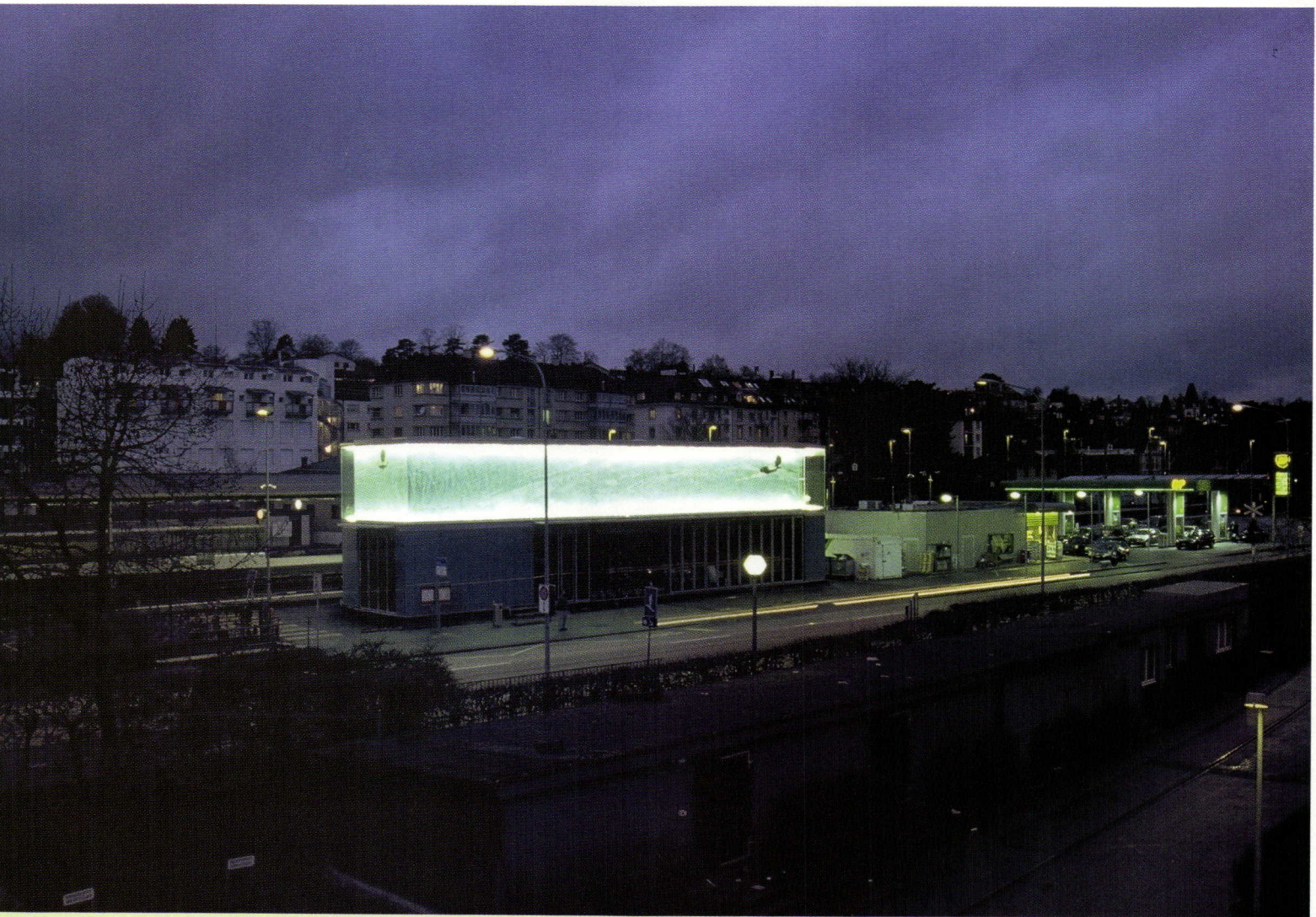
Details developed by the architects lighten the boxy structure, which comprises steel-tube columns and concrete slabs. The envelope is double-skinned, with insulated metal panels that are inset slightly from the exterior of the glass curtain wall on the second floor, underscoring the building's dual functions.
