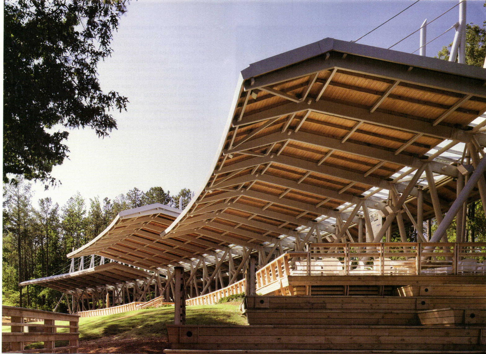
Opposite the performance pavilion is the crescent seating area, which employs the same structural vocabulary. Rawn placed the building on a natural rise in the landscape, providing VIP concertgoers with unencumbered views of the stage.
