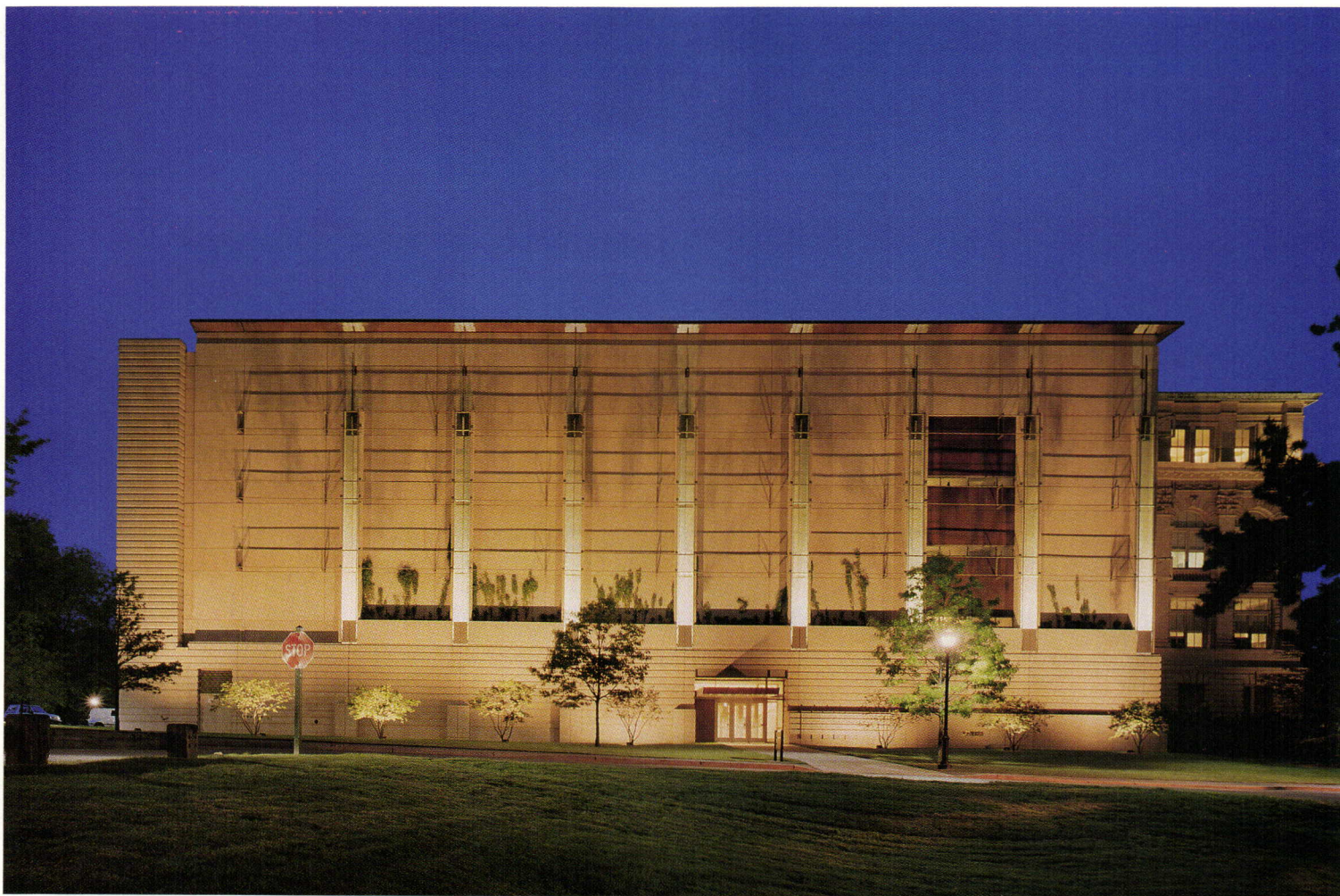
The entry sequence is through a deeply carved portal slightly off-center-right that is overhung by a simple copper canopy echoing the form of the cornice. The entrance bypasses mechanical spaces to the north and directs people through a cherry-paneled lobby to the elevators, which serve both the old and new buildings.
