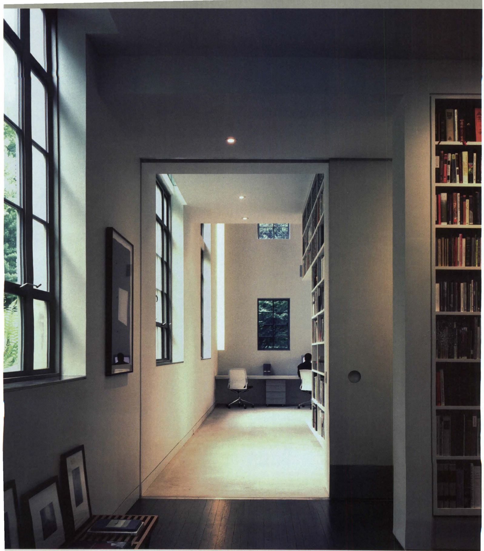
The division between the living and work wings of the house is marked by a sliding door and a change in flooring from wood to concrete.
