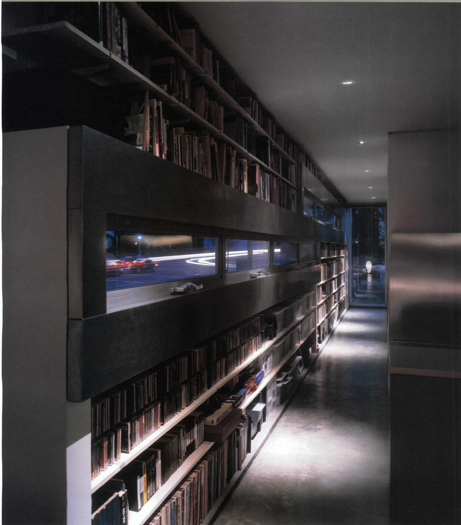
To allow the bookshelves and ribbon windows to be flush on the interior required the construction of two walls.
