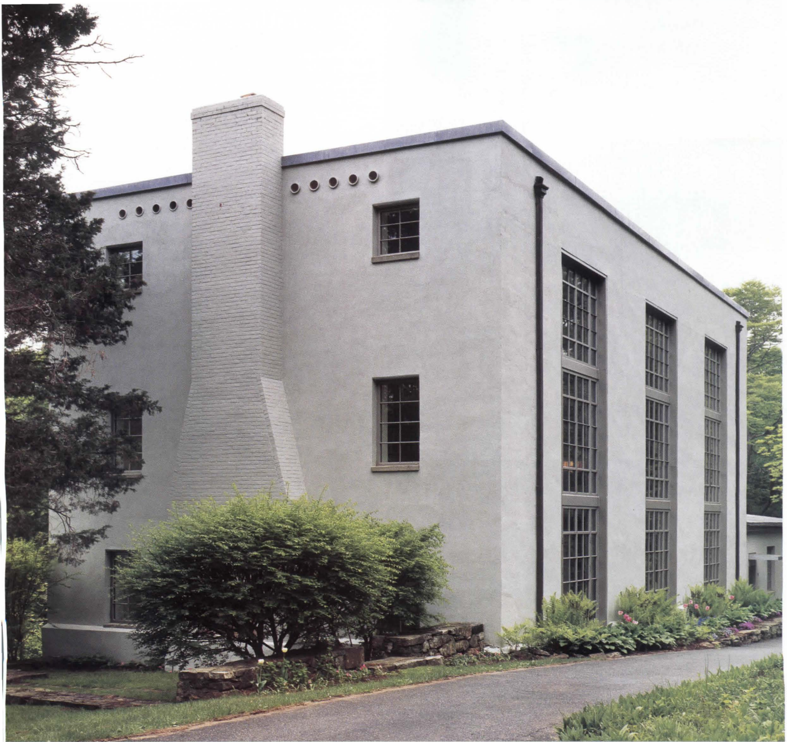
The north façade is dominated by gridded, three-story windows (facing page, left, and above), while the south façade (facing page, right), which parallels the road, is predominantly opaque.
