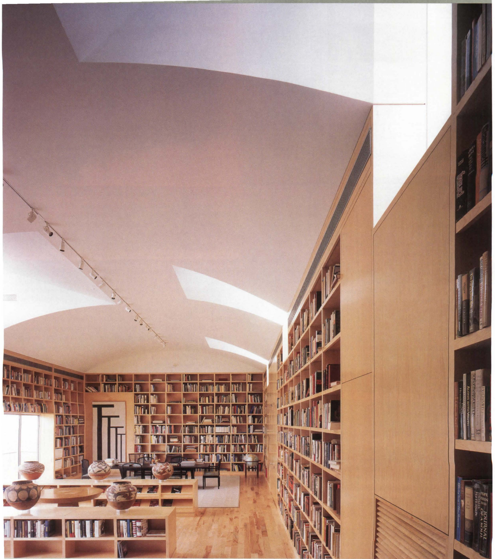
Clerestory windows function as skylights; the eastern openings are incised into the arched ceiling at a steeper angle than those on the western side.
