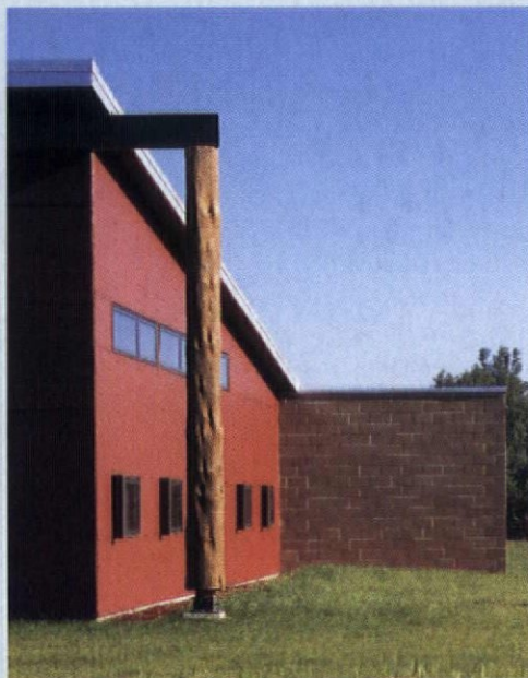
Rods and turnbuckles help brace open façades (left), and rough-hewn columns support the southern beam line (center). High-bay windows flood the whitewashed interior with daylight, and a lower rank of windows offers views to occupants seated in private and open offices (right). The casework is made of formaldehyde-free particleboard.
