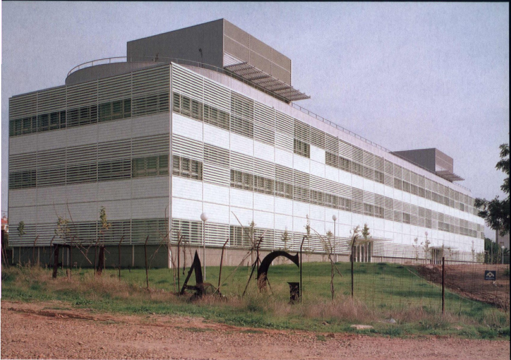
Graduate classrooms and administrative facilities are housed under a heat-absorbing grass roof at the University of Extremadura in Mérida, Badajoz, Spain. Part of a campus expansion toward the River Guadiana, the three-story, 300-foot-long building (above) is encased in a skin of lattice-work that filters natural light and surrounded by a ring of trees that when mature will serve as a natural layer of protection against the sun. A running track on the roof wraps the edge of the grassy zone and two small penthouses, which hold lounge areas for the staff (facing page).
