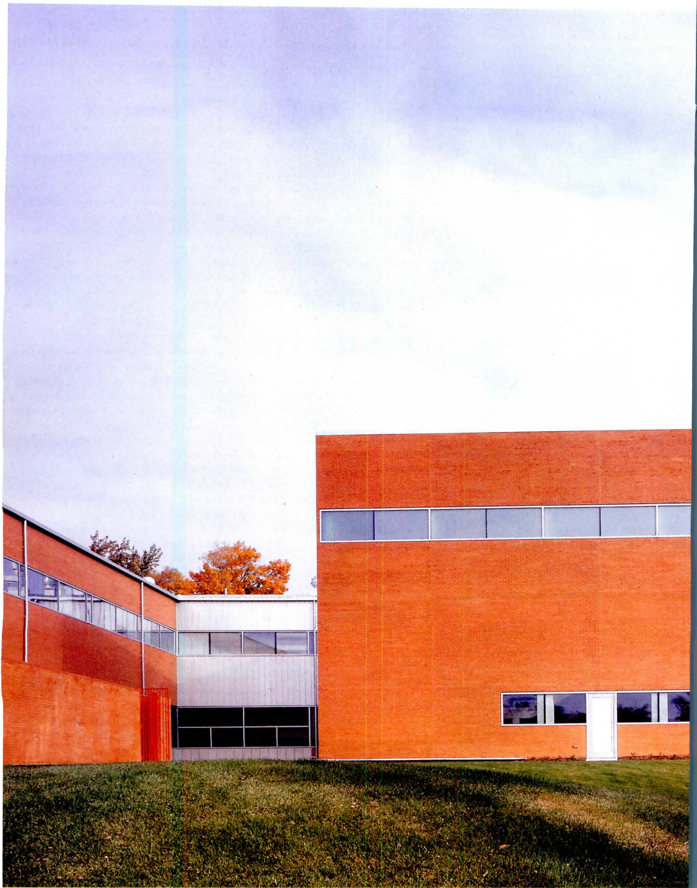
A courtyard and sculpture garden establish preliminary connections with nearby campus buildings and grounds (above). Steel panels, brick veneer, and ribbon windows express interior functions and modulate the tightly drawn building envelope.
