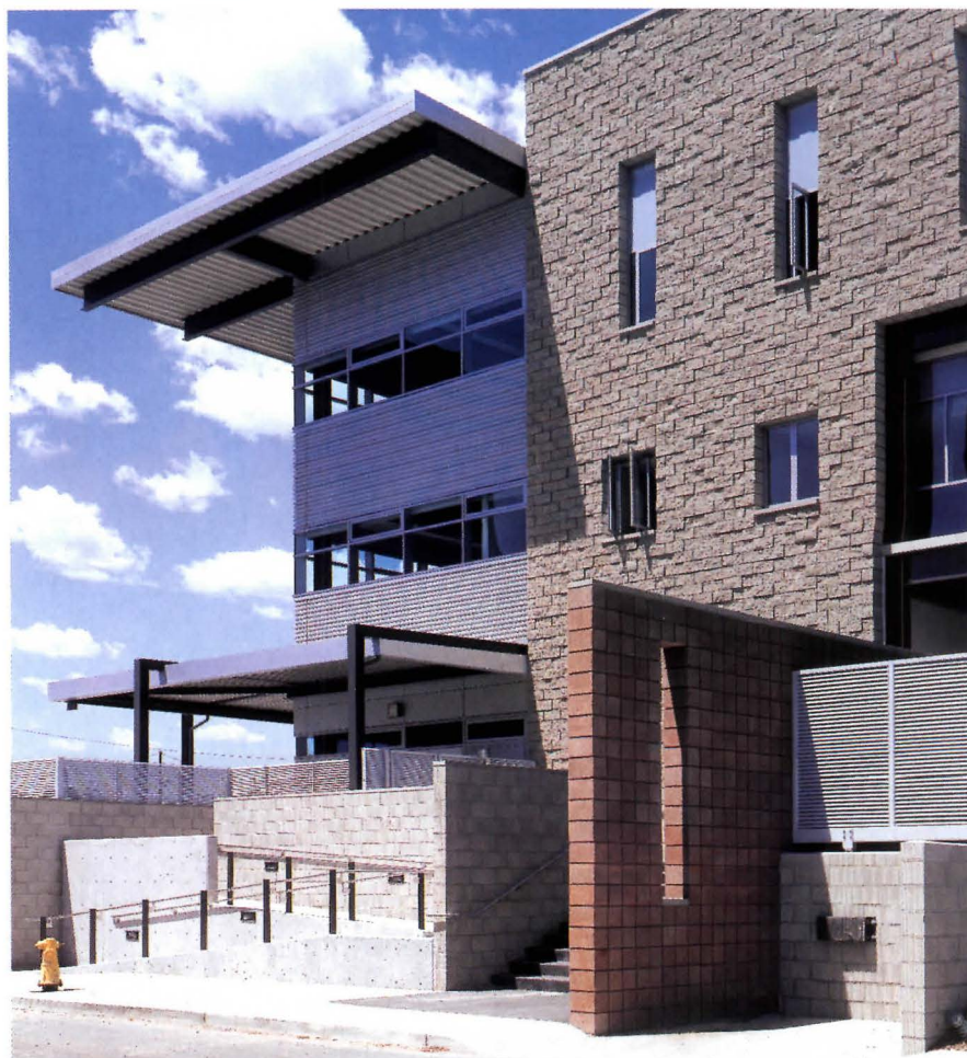
Located at the southwest periphery of campus, the staging building features a "head" of split-face concrete block to the north and flanks of metal cladding with deep overhangs (top) that meet a wall section of concrete block facing Wilshire Boulevard to the south (bottom).
