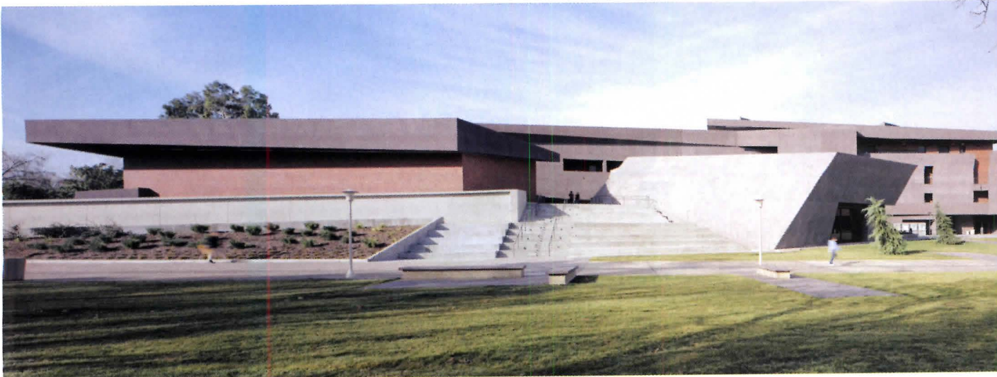
In color and form, the art center suggests the canyons and mesas of a nearby mountain range and the arroyo that runs through the campus. The connected buildings are essentially rectangular forms arranged with several overlapping and skewed structural grids.
