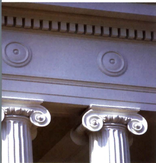
Forming a quad with buildings from the 1950s and the early 1970s (including Burden Auditorium by Philip Johnson), the Spangler Center brings a fully detailed Ionic order, replete with dentils and echinus (above left), to the Harvard Business School campus.
