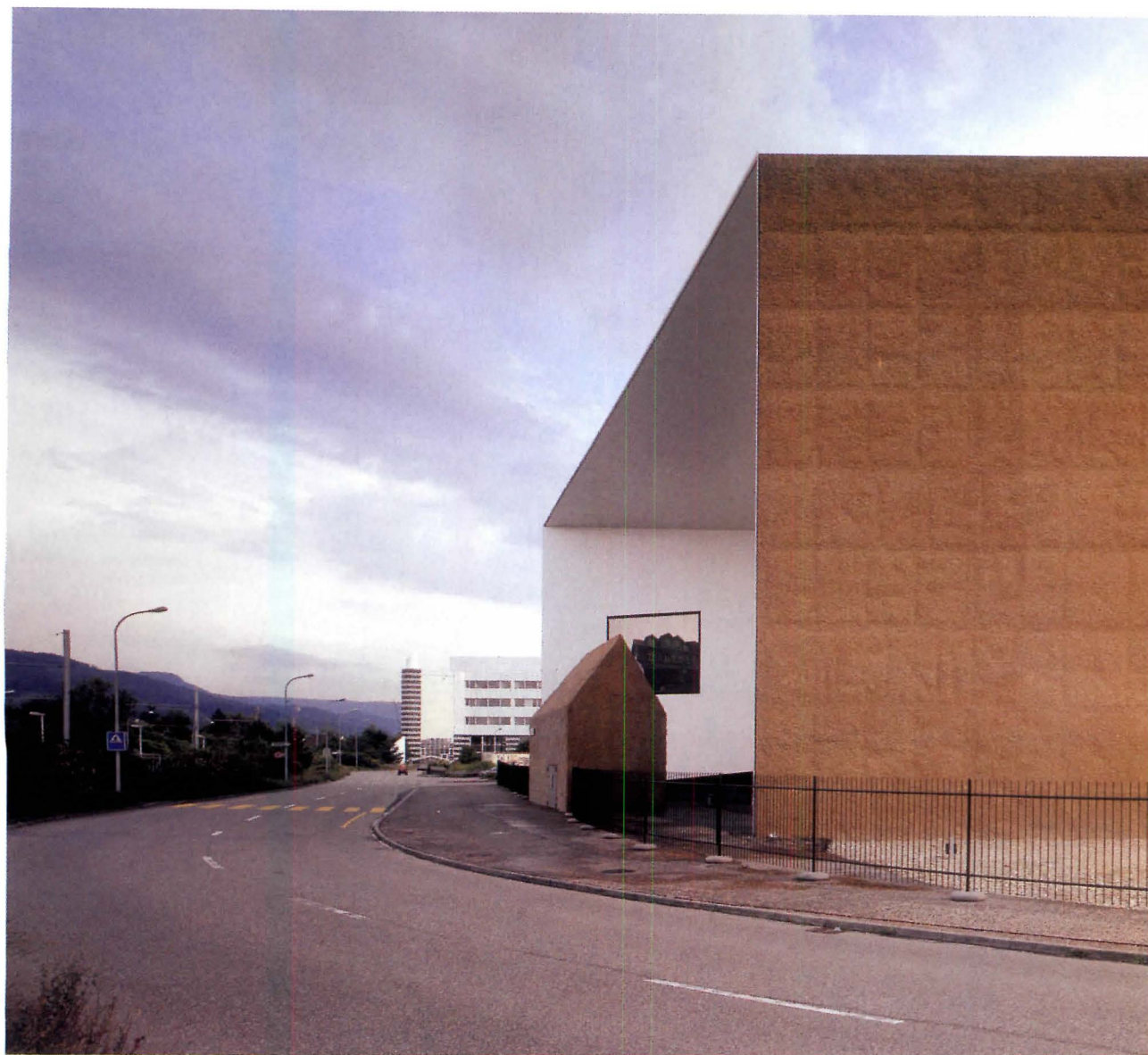
A forecourt facing Emil-Frey Strasse comprises an indented polygonal façade on which two 473-square-foot LED screens are mounted. Art pieces commissioned by the Schaulager appear on the screens, altering the façade as they are changed over time.
