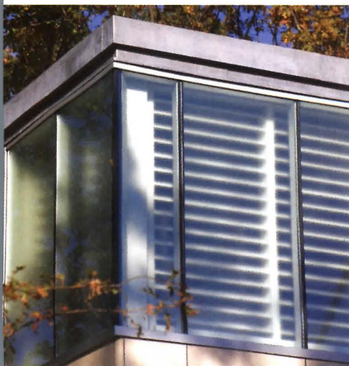
A glass-enclosed staircase follows the natural contour of the hill on which it sits (opposite, right). Lightweight ceramic tiles echo the limestone of the existing museum, and a clerestory of diffusion glass with louvers controls natural lighting in the new gallery (above, left).
