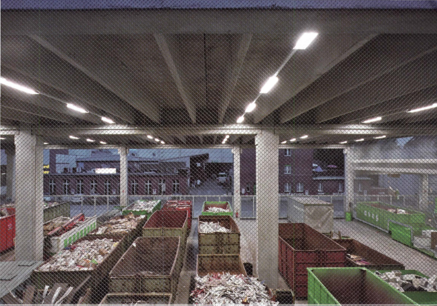
Containers of sorted metals, paper, plastics, and glass waiting to be shipped or trucked to production-side customers are held in Maag's storage depot (above). A stairway wrapped in galvanized metal mesh and cantilevered from the prefabricated concrete structure leads to a rooftop garden and parking (facing page).
