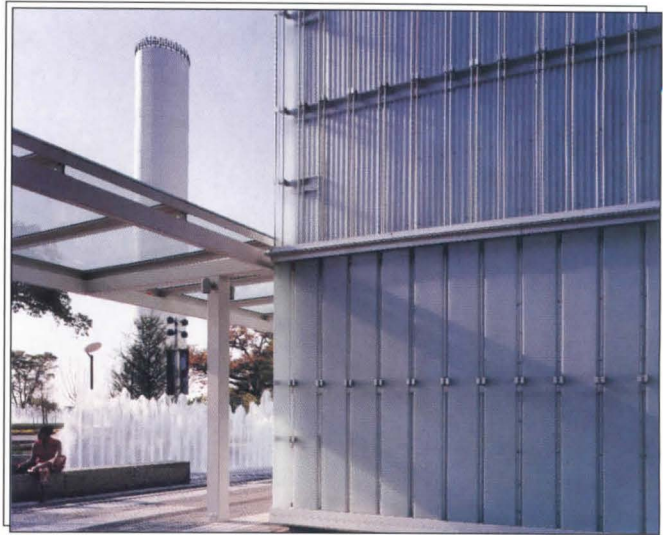
At street level, the Shaw Center's glass channels are turned inward and sandblasted; higher up, translucent channels allow views of opaque art-gallery walls, which are installed adjacent to the glass rainscreen.
