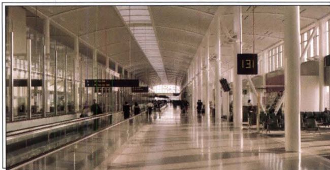
The toroidal roof of Toronto's new terminal (top) crowns the departures hall. Passengers follow skylights that line each pier building (above) to find their gates.
