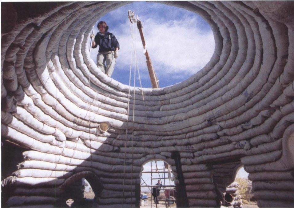
NADER KHALILI'S SUPER ADOBE, CONSTRUCTED FROM "THE MATERIALS OF WAR."
