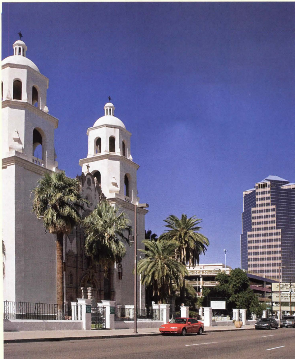
St. Augustine Cathedral's façade (at left), created between 1897 and 1928, was kept during a 1960s sanctuary overhaul.
