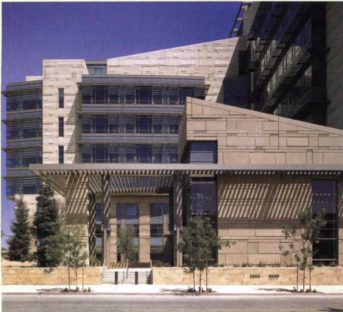
U.S. Courthouse, Fresno, Calif. (honor award: architecture, completed projects)—Gruen Associates and Moore Ruble Yudell
