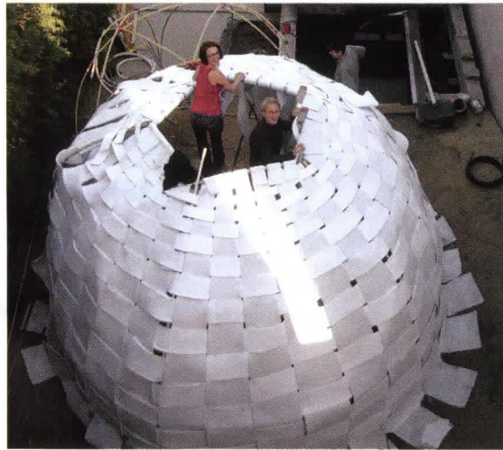
The fabrication team learned the art of bamboo lashing to hold the structure's tension frame (far left) together, but ended up using duct tape, which proved easier to work with. At left: the installation nears completion.
