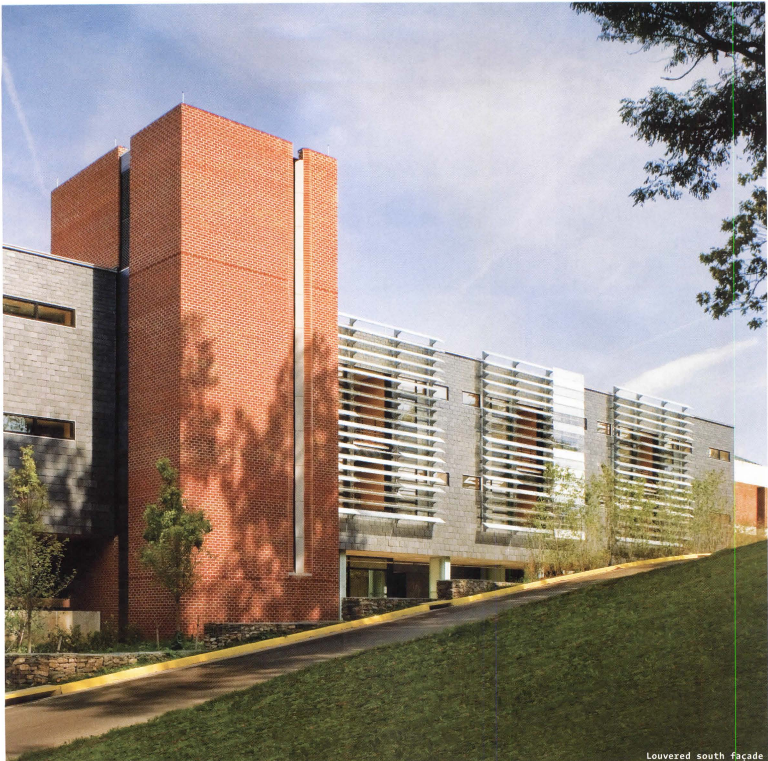
Louvered south façade
