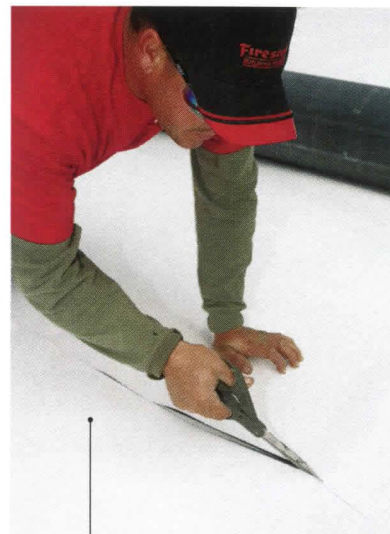
Firestone's latest EPDM rubber membrane, RubberGard EcoWhite , adds 60-mils of membrane to the roof with a simple roll installation. It has a solar reflectance of .80 and a solar reflectance index of 99, when tested in compliance with the Cool Roof Rating Council. • 10', 16'-8", 20', or 25' widths • www.firestonebpco.com • Circle 106
