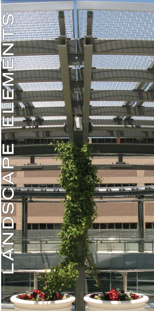
Surrounding an open air atrium on the roof of this new medical facility a circular overhead trellis uses tapered greenscreen® panels.
