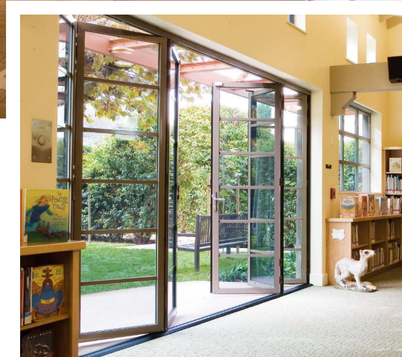
Palo Alto Children's Library Palo Alto, CA NanaWall Aluminum Framed Folding System SL45 Architect: Architectural Resources Group
