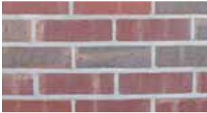
Figure 6. Extruded brick, Type FBS, with a velour texture
