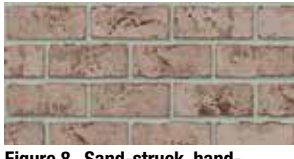
Figure 8. Sand-struck, hand-molded Type FBA brick
