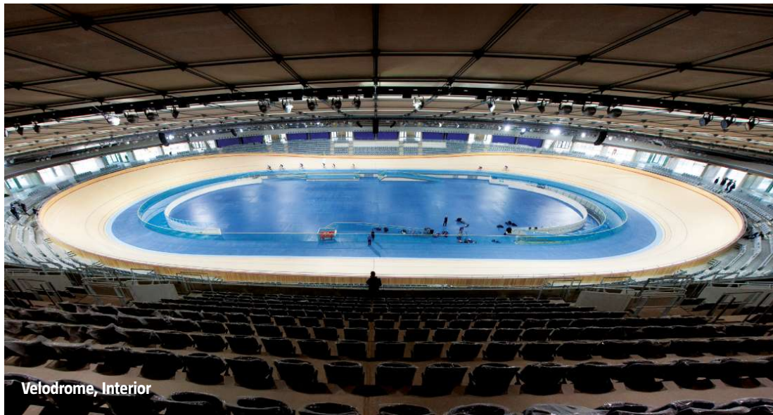
Velodrome, Hopkins Architects
