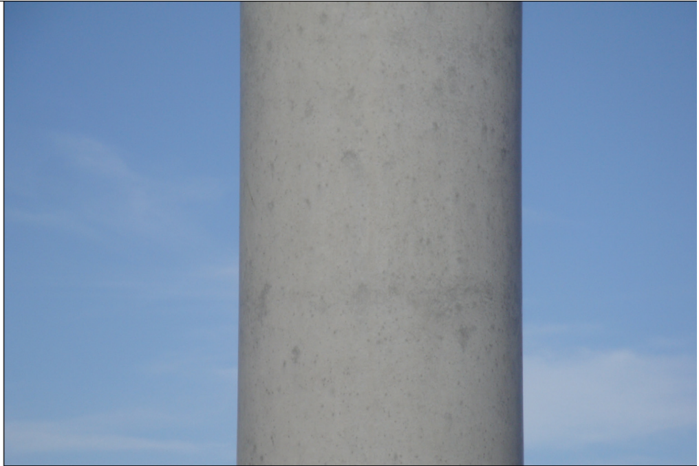
Seam-free forms provide the desired finished look without having to sand, grind or otherwise re-finish the surface to remove or patch spiral seams, rust, saw marks, bug holes or other surface imperfections common with other forms materials.
