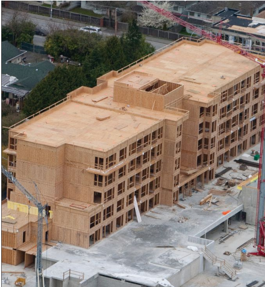
Wood-frame construction has shown strength, longevity and stability, and is widely considered economical, with low material costs, reduced construction time, and availability of resources and labor. Photo: Stephanie Tracey
