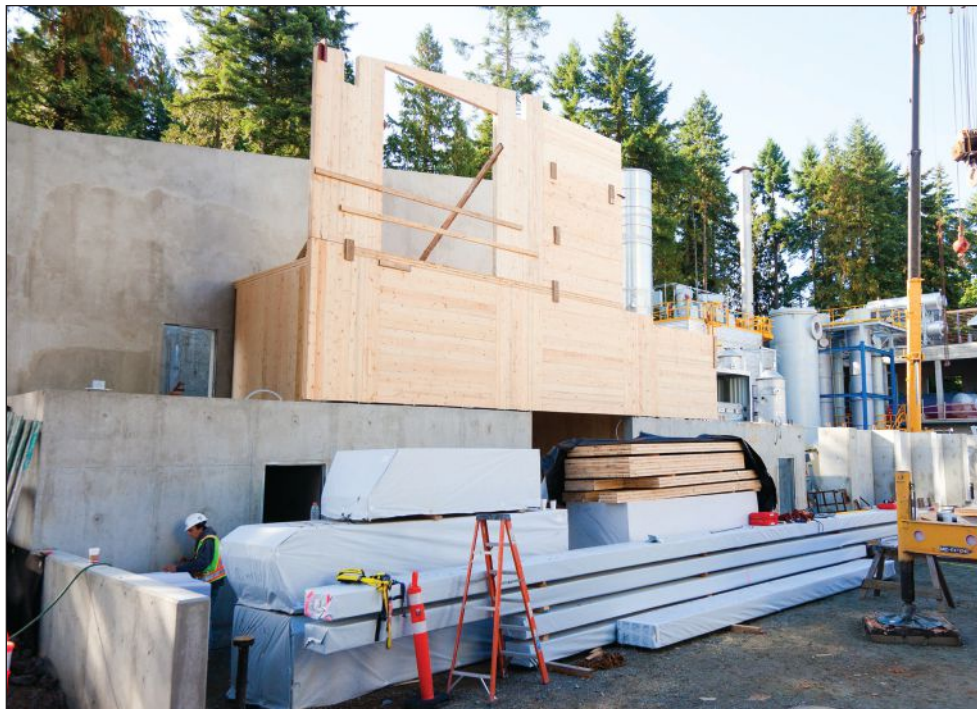
Wood should be stored and wrapped properly on a construction site. Photo credit: KK Law
