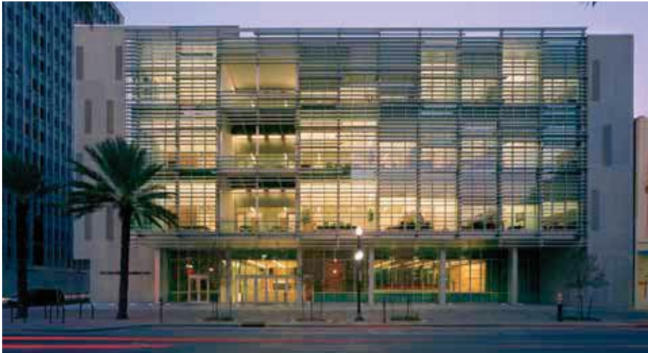
For this new lab and incubator office building in New Orleans designed by Eskew+Dumez+Ripple, glazed areas are heavily shaded or recessed into punched-out openings. The opaque walls are made of a hybrid system of thin precast concrete on a light-gauge steel frame, shop-applied with continuous spray-foam insulation and weather barrier. (Photo by Timothy Hursley, courtesy Turner Construction)
