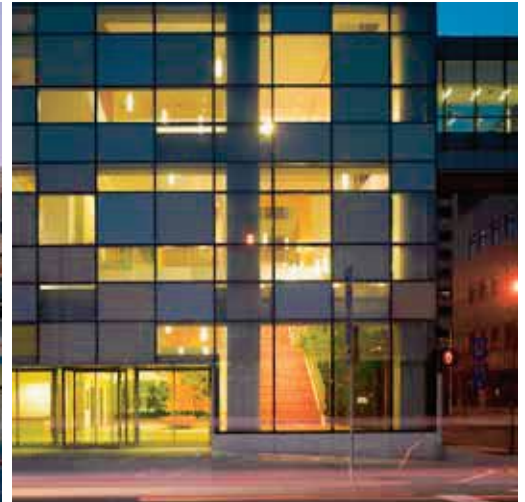
For 55 Park Street, a clinical lab building in New Haven, Connecticut, Behnisch Architekten and executive architect Svigals + Partners developed a curtain-wall façade of translucent and reflecting panels dictated by the lab layout within and energy efficiency goals. The insulated, high-performance curtain wall was systematically applied in order to temper the indoor environment in response to both façade orientation and diverse interior requirements. (Photo by Roland Halbe)
