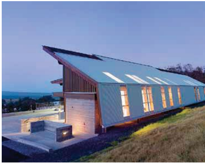
Hawaii Prep's Energy Lab in Kamuela, Hawaii, has an energy-efficient enclosure with a traditional tropical three-pitch roof design that shades a lanai area on the south-facing exposure and carries mauka (mountain-side) winds moving across the roof to create an augmented vacuum in the broken peak. Local lava rocks were added as aggregate to the poured concrete wall. (Photo by Matthew Millman, courtesy Flansburgh Architects.)
