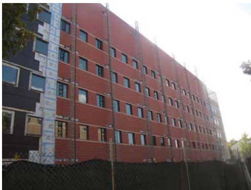
The SmithGroupJJR designing a project that is targeting LEED platinum certification as sustainability and energy efficiency was a top priority. The team designed a pressure equalizing terracotta rainscreen cladding system provided by Shildan in conjunction with an R30 thermal envelope for optimum energy performance.
