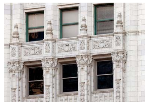
New windows shown in the bottom row.
