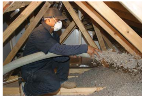
While a form of cellulose insulation was used in Thomas Jefferson's Monticello, the modern iterations of the material is often made from recycled newspaper and treated with fire retardant chemicals. Credit: Photo courtesy of Bonded Logic Inc.
