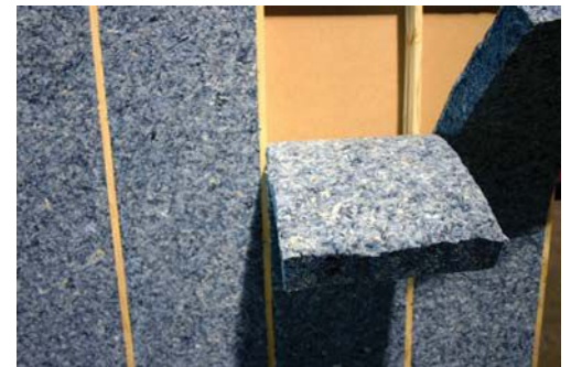
Batt insulation made of recycled cotton and denim creates tiny air pockets that stem the flow of thermal energy. Oversized batts produce a friction fit between studs in wall cavities. Credit: Photo courtesy of Bonded Logic Inc.
