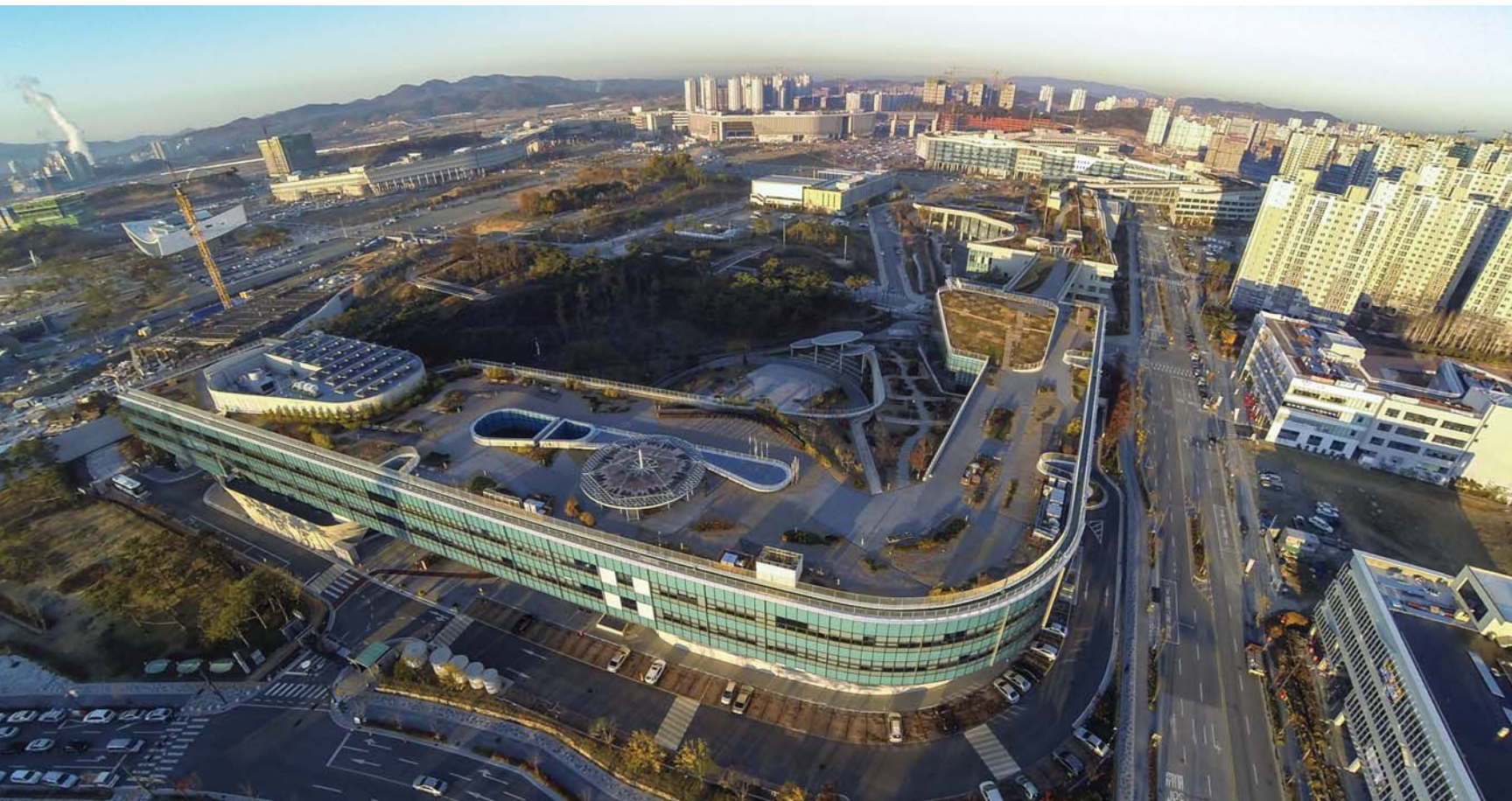
Previous spread: A diagram of the circulation and transportation infrastructure surrounding the Sejong City government complex. Top: Infrastructure at street level is complemented by a parallel system of footpaths and gathering areas on the landscaped roofs of the government complex. Above: Far more than your typical green roofs, these have a distinct public role and identity within the new urban environment.
