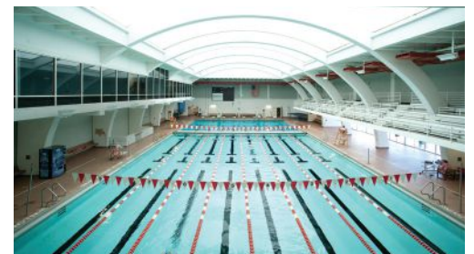
The Donald D. Dedmond Center Natatorium, Radford University, Radford, VA is an example of how advancements to the membrane to can provide translucency and insulating capabilities.
