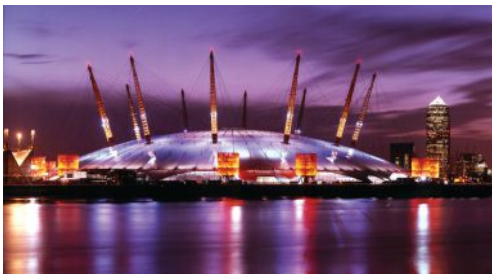
The O 2 , in Greenwich England, is the largest cable-supported domed structure in the world.
