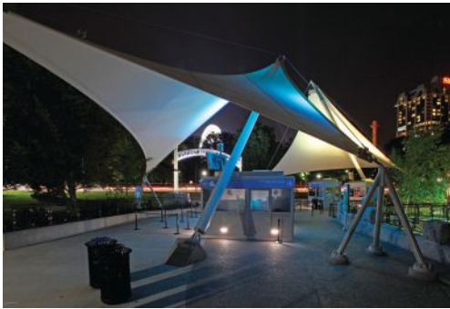
Two sail-shaped PTFE membrane canopies create a dramatic and signature look at the entrance of the Hornblower Niagara Cruises.
