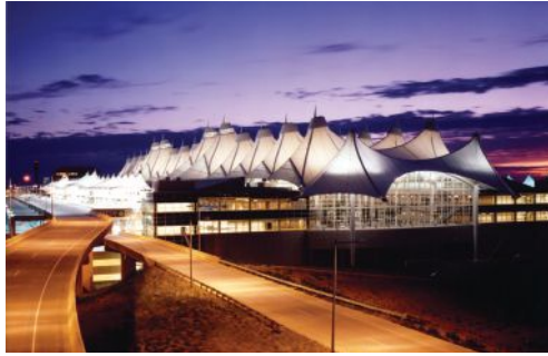
Denver International Airport's tensioned fabric membrane roof pays homage to the region's iconic Rocky Mountains.
