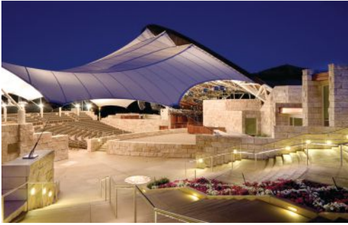
With tensile construction, biaxial forms can be readily achieved as they flow naturally from the materials installed in tension.
