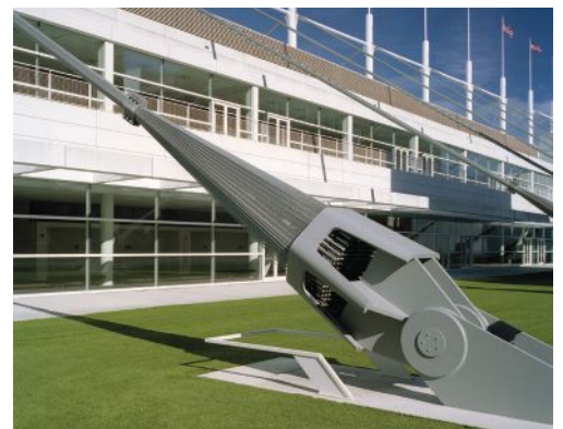
Caption: Bundled cable systems are massive and impressive structures themselves and allow efficient means for creating dramatic effects.
