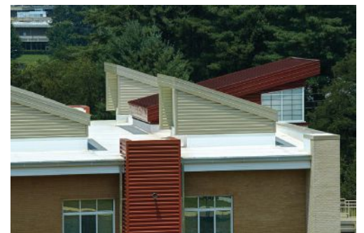
Metal roofing materials are often selected due to their durability and low maintenance. Photo courtesy of Petersen Aluminum
