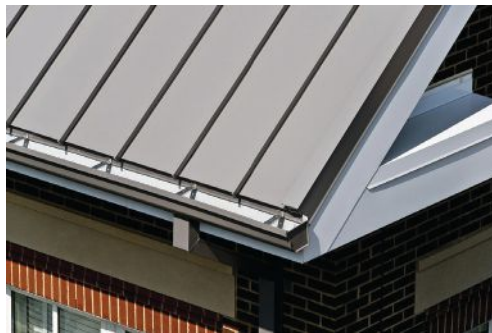
Standing seams are traditional metal roof designs with concealed fasteners. Photo courtesy of Petersen Aluminum
