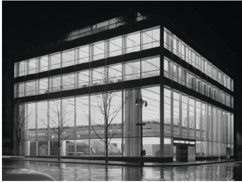
The Manufacturers Trust Company Building is a striking example of a luminous, thermoformed ceiling. The New York City Landmarks Preservation Commission says, "Corrugated 'paper thin vinyl sheeting,' hung from T-shaped metal channels, gave the ceilings an uncluttered directional character. With none of the lighting fixtures visible, it could easily be seen from both streets and reads as a floating, illuminated grid." The building was designed by Skidmore, Owings & Merrill and completed in 1954. Design: SOM / Photo: © Ezra Stoller/Esto
