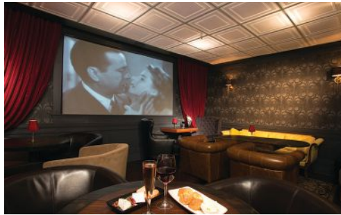
Ceiling panels with classic detailing complement the theme of the moving screening room in a Noir Lounge in San Francisco. The thermoformed translucent material "creates a gentle glow and avoids glare on the screen," according to architect Gi Paoletti of G. Paoletti Design Lab. She adds that dimmable LED lamps above the luminous ceiling avoid the need for pendant light fixtures that would block patrons' view. Design: G. Paoletti Design Lab / Photo: Stuart Locklear
