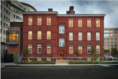
When specifying windows it is very important to take into consideration both rough and masonry openings. Photo courtesy of Chad Holder Photography
