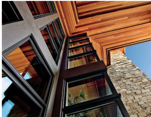
The frame description should include the window style and shape, both interior and exterior finishes, basic dimensions such as the thickness and depth of the frame, and the use of certified wood, if required. Photo courtesy of Blackstone Edge Studios
