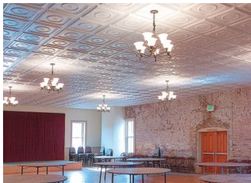
The brick walls and hard surface floors of this meeting hall required a ceiling with good sound absorbing properties. For remodeling projects, thermoformed ceilings are also light weight to minimize loads on existing structures and can be installed beneath existing sprinklers. Photo: Ceilume
