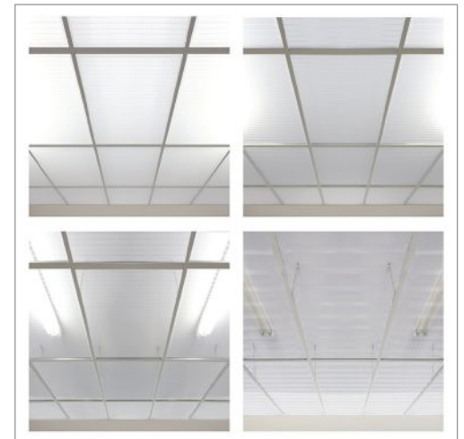
Translucent panels (top left) create the most even light distribution. Frosted panels (top right) hint at what is above the ceiling. Transparent panels fully disclose what is above the ceiling whether above-ceiling lamps are on (bottom left) or off (bottom right). Each ceiling style will scatter light differently; some display patterns of highlights and shadows or sparkling refractions that become animated as one moves through a room. Photo: Ceilume
