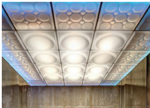
This cloudscape was created with two styles of billowing translucent panels. The relief projects downward on one style and upward on the other to enhance the interplay of shadows and highlights. LEDs above the ceiling can be dimmed to adjust from high noon to the warmer tones of late afternoon. The drop-out panels are installed beneath fire sprinklers. Design: Emma Davis Interior Design / Photo: Ceilume
