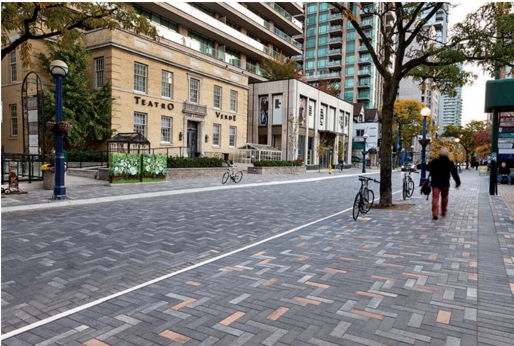
Paving stones laid from building front to building front helped revitalize Toronto's trendy Yorkville Avenue shopping district.
