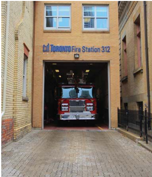
The paving stones installed outside the Fire Hall on Toronto's Yorkville Avenue held up for more than 40 years of heavy traffic from fire trucks weighing more than 35 tons.
