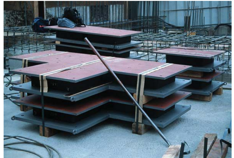
At Lucky Goldstar Kangnam Art Hall in Seoul, South Korea, this typical acoustical isolation system detail features lateral isolation pads and a reinforced concrete grid within the structural steel system. Photo courtesy of SOM
