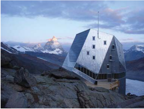
Built within the jagged mountains of the Swiss Alps, the Monte Rosa Hut has its own water supply provided by the mountainous terrain and was designed to blend with the surroundings and minimize the facility's exposure to wind and snow. Photo courtesy of Holcim Foundation and Wikimedia Commons.
