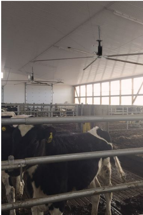
Series of I-Class fans used in dairy barn for ventilation and destratification.
