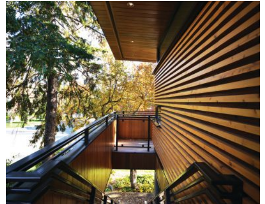
Western Red Cedar’s scientific name is Thuja plicata . The name is derived from thujaplicin, a chemical substance that is found in mature trees and serves as a natural fungicide, thereby preventing the wood from rotting. Photo courtesy of Houry Avedissian.
