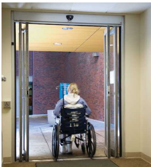
Most auto-swing and auto-slide systems have adjustable control of the hold-open time as well as adjustable time-delay closing, ranging from two seconds up to 30 seconds.
