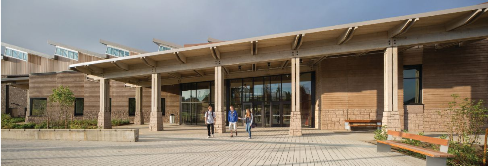
Because the buildings needed to last at least 75 years, the architecture firm of DOWA-IBI Group Architects decided on a proven, durable wood siding. Photo courtesy of Josh Partee.
