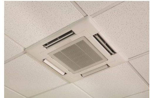
A 4-way ceiling-recessed cassette can be used to provide a more spacious feel.
