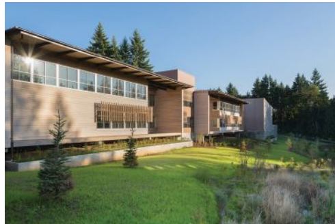
The use of Western Red Cedar helped reinforce the desired modern Cascadian aesthetic. Photo courtesy of Josh Partee.
