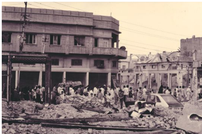
The demolition of Baghdad's Haifa Street in 1981
