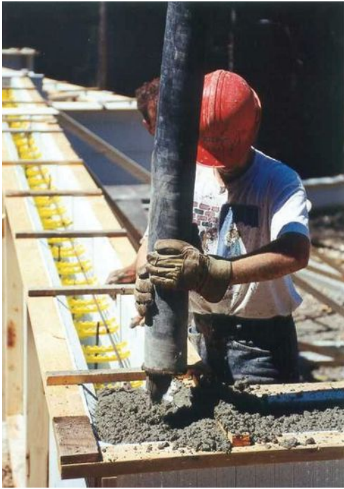
Concrete being pumped into an ICF wall. Photo courtesy of Quad-Lock®.
