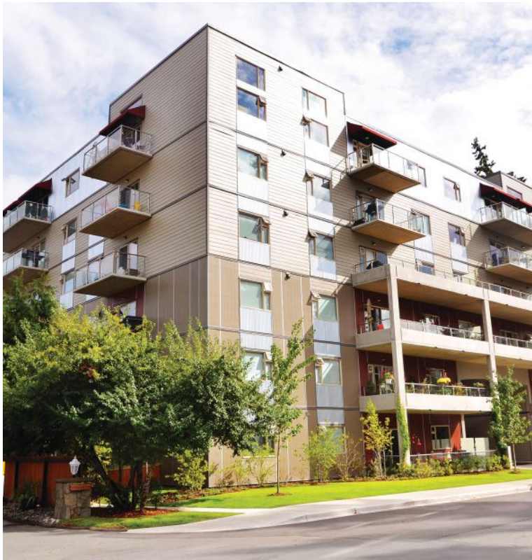
Apartment building built using Insulating Concrete Forms (ICFs). Photo courtesy of Nudura®
