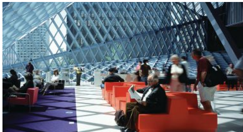
At the Seattle Central Library, the design of a steel diagrid eliminates 90 percent of the aluminum that would typically go into a façade mullion system. Photo courtesy: Pragmesh Parikh/MKA
