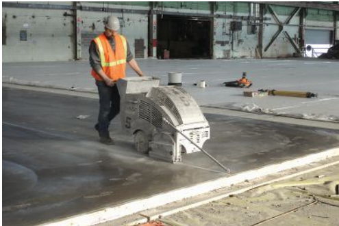
Sawcutting a control joint on a new slab.
