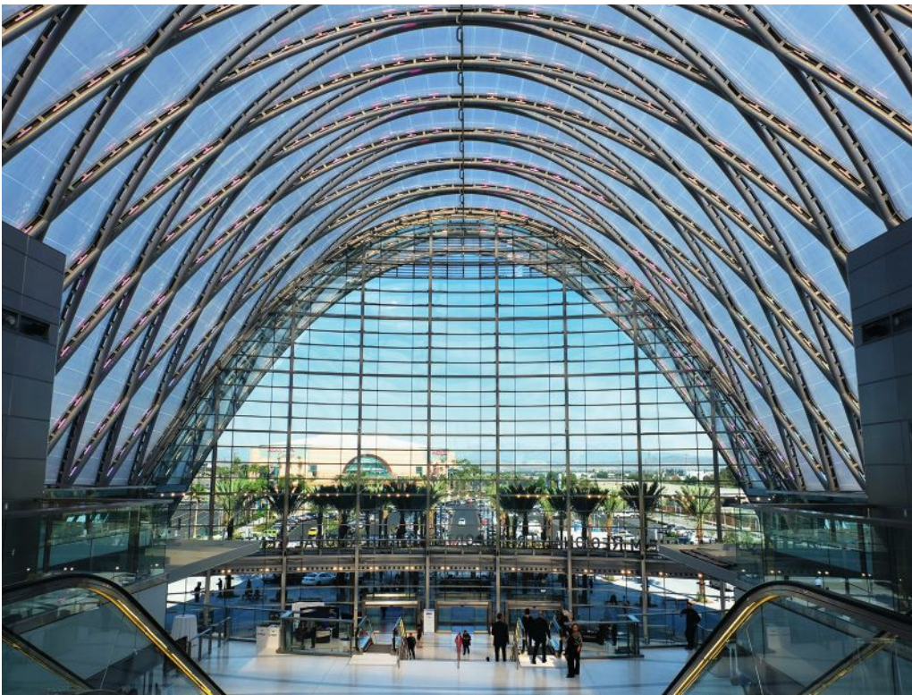
Long spans, curved steel members and abundant natural light highlight the new Anaheim Regional Transportation Intermodal Center in Anaheim, Calif., which won a 2015 AISC IDEAS 2 Award and achieved LEED Platinum certification. Photo courtesy: Thornton Tomasetti, Inc.
