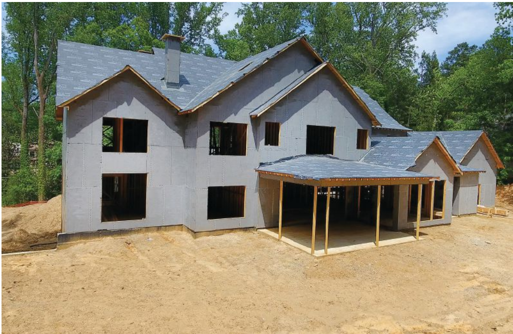
Integrated air and water barrier system application
