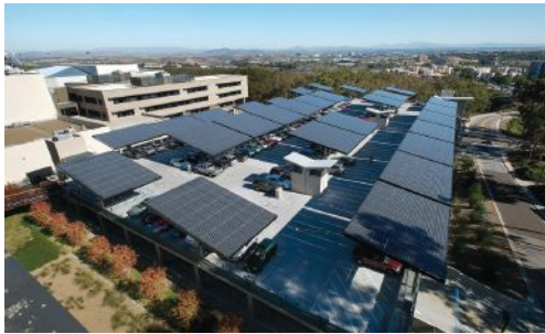
Hopkins Parking Structure, San Diego, CA Hopkins Parking Structure at the University of California San Diego campus uses photovoltaic cells for parking lot canopies and high albedo concrete in the driving lanes to help reduce the urban heat island effect. Photo: University of California San Diego
