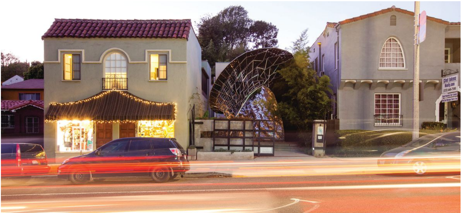
A 2011 street view of Bloom, which displayed the many scales of hyperbolic paraboloids for lightweight strength.
