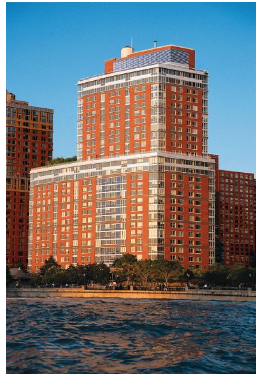
The Solaire, New York, NY The $120-million Solaire in lower Manhattan's Battery Park City stands 27 stories tall with 293 rental units. A reinforced concrete structural system was chosen in large part because its thermal mass moderates daily temperature swings and reduces energy needed for heating and cooling. Among its many environmental benefits, the building is designed to consume 35 percent less energy, a savings that is potentially worth 14 points toward the LEED Energy and Atmosphere credit. Design Architect: Cesar Pelli & Associates Architects. Photo: www.concretethinker.com
