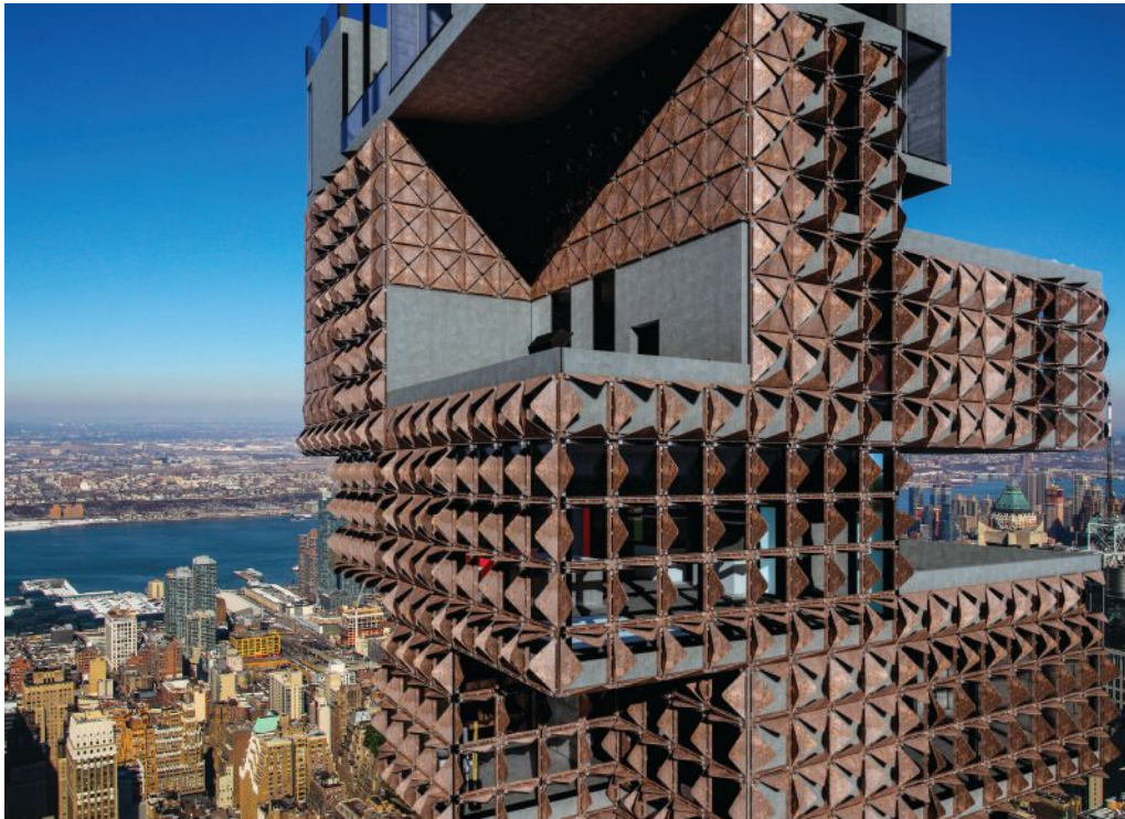
Three-dimensional prototyping and modeling can help create buildings that are better designed, easier to construct and safer to use, as shown here in the WPF CAD Shared Tower. Photo credit: Jan Philipp Wotschke; Courtesy of Vectorworks, Inc.
