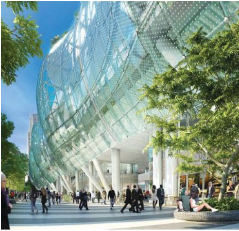
A performance-based design approach for San Francisco's Transbay Transit Center enabled Arup to meet two-hour fire resistance requirements by filling the large diameter hollow sections with concrete. Photo courtesy Transbay Transit Center
