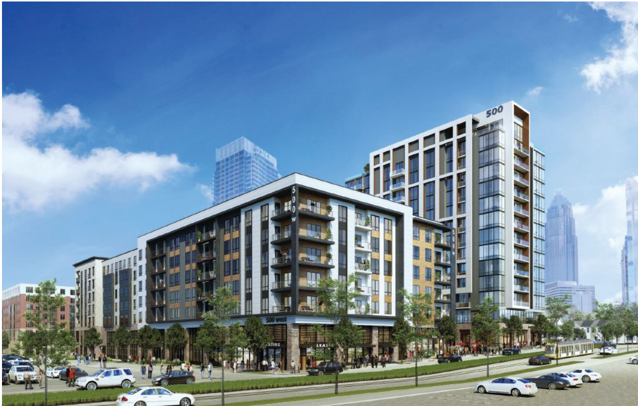
Construction is expected to begin this year on 500 West Trade, a 354-unit Charlotte, N.C. apartment community, that wraps a 6-story mid-rise podium wood frame structure around a 14-story steel and concrete tower. The hybrid design allows a more diverse rent structure, with the mid-rise portion offering more affordability and unit density. The location is an abandoned 2.8-acre site in downtown Charlotte. Image courtesy of Dwell Design Studio
