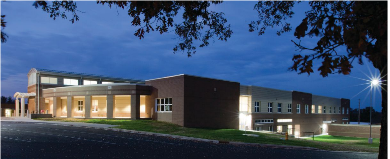
Richardsville Elementary School in Warren County, Kentucky, is the nation's first zero-energy school. Architect and photo credit: Sherman Carter Barnhart. MEP Engineer: CMTA, Inc. ICF System: Nudura.
