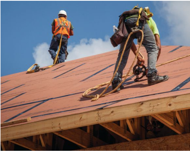
Integrated sheathing with built-in air and water barriers helps streamline construction and reduce the chance of water penetration during a high-wind event, if the roof covering is blown off.
