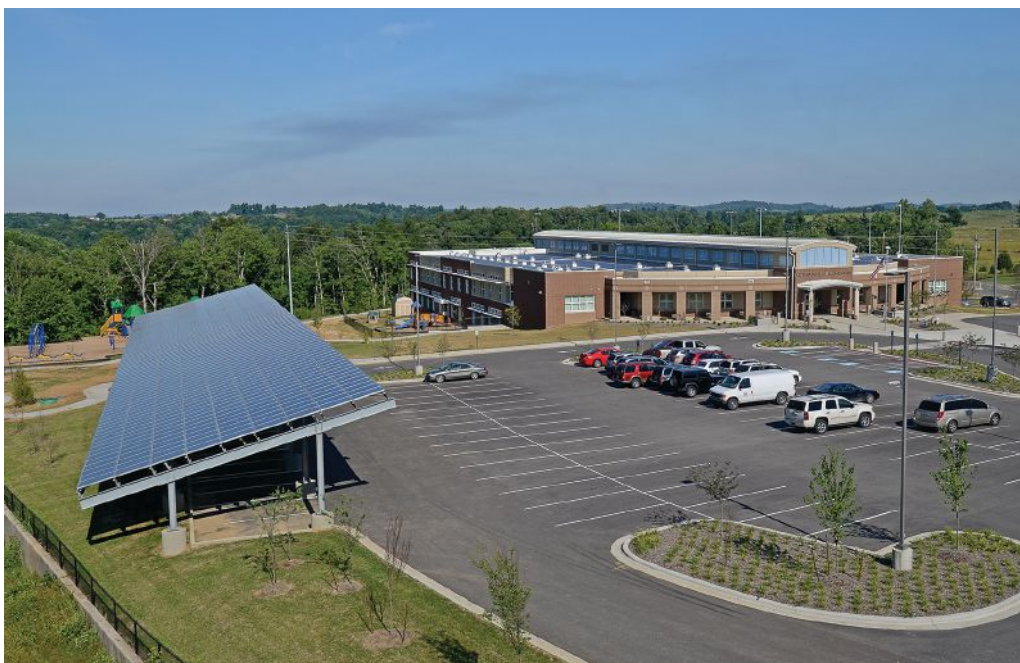
Richlandville Elementary School is so energy efficient that it generates enough energy to sell back to the electric utility. Photo courtesy of CMTA, Inc.
