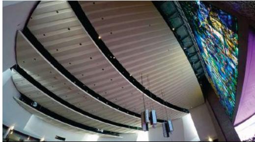
Drywall: Winning Project United Methodist Church of the Resurrection Leawood, Kansas
