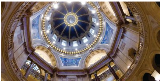
Interior Plaster: Winning Project Minnesota State Capital Repairs, Restoration and Preservation St. Paul, Minnesota
