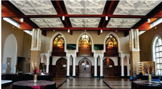
Ceilings: Winning Project St. Mark Coptic Orthodox Church Troy, Michigan
