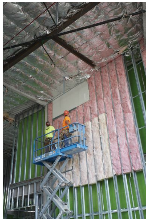
The construction of framing and gypsum board partitions is fast, efficient and very flexible. Photo courtesy: USG.
