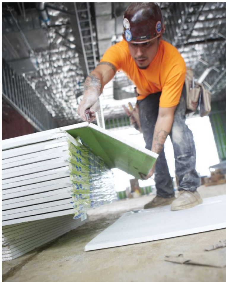
Glass-mat interior panels offer enhanced protection against water and air infiltration, and is available as a abuse-resistant product, with fire protection and acoustical benefits. Photo courtesy: USG.
