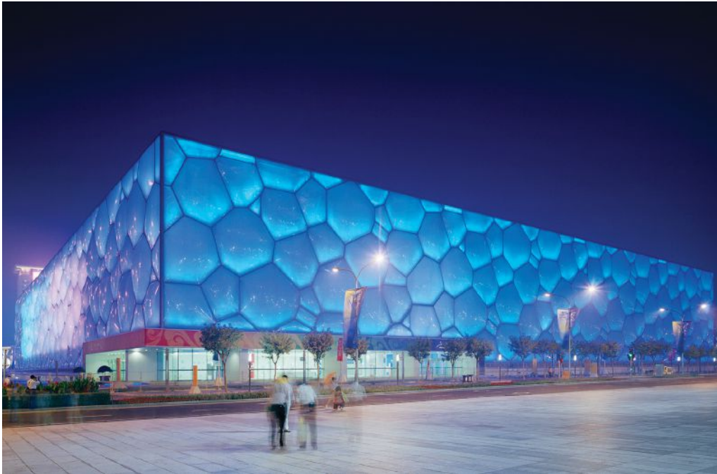
The single largest application of ETFE cladding technology to date is the National Aquatic Centre (The Watercube) with 1,076,391 ft 2 in Peking. (Image © Werner Huthmacher)
