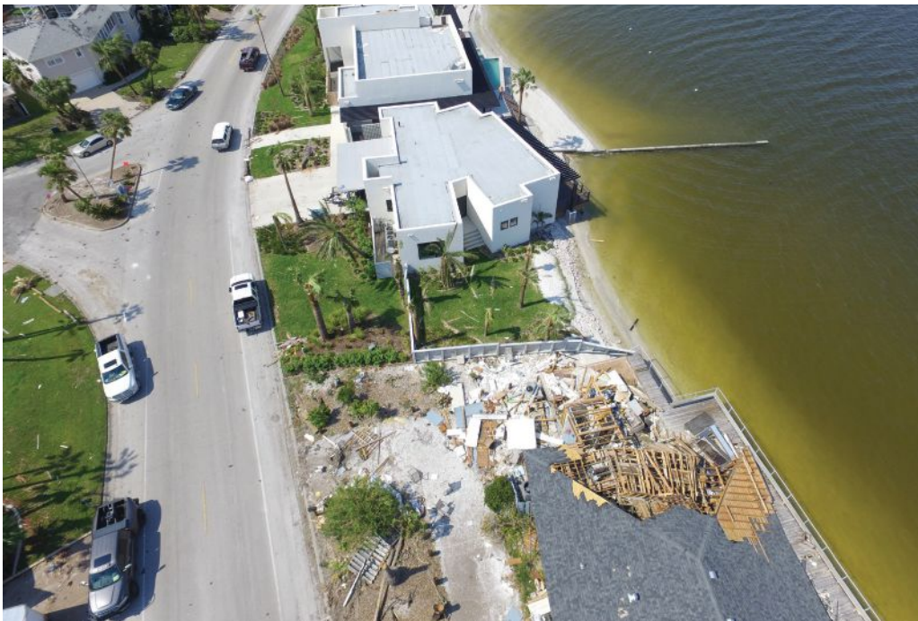
Despite the destruction from Hurricane Harvey, the ICF building remains intact.
