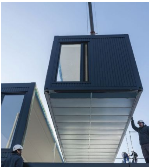
One technique for creating temporary pop-up architecture is to use modular components such as trailers or shipping containers. Photo courtesy of: Christoph Merian Stiftung, Basel
