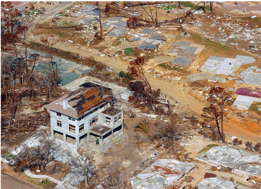
This image shows the devastation from Hurricane Katrina, with sole resilient building (ICF construction) standing.
