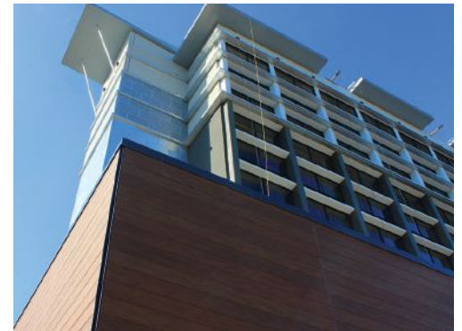
Extruded Aluminum Trim paired with multiple siding products including a commercial rainscreen fiber cement and others on a Holiday Inn and Suites.
