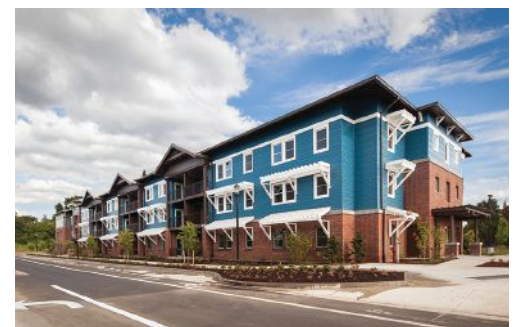
Since we relax and sleep at home, it is important for sound mental health that noise is mitigated in our personal space. Residential noise issues can arise from floor/ceiling footfall, party (demising) walls, plumbing, HVAC and elevators and/or trash chutes. Orchards at Orenco | Architect: Ankrum Moisan Architects, Inc. | Photo: CBPhotography & Designs
