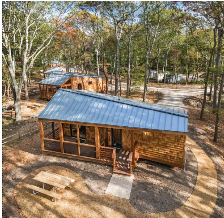
Roofs are clad in galvalume from Petersen Aluminum Corp.
