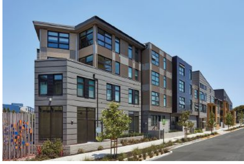
Located on the border of Emeryville and Oakland, this multifamily housing development on 3900 Adeline Street includes 91 residential and 10 work/live rental units.
