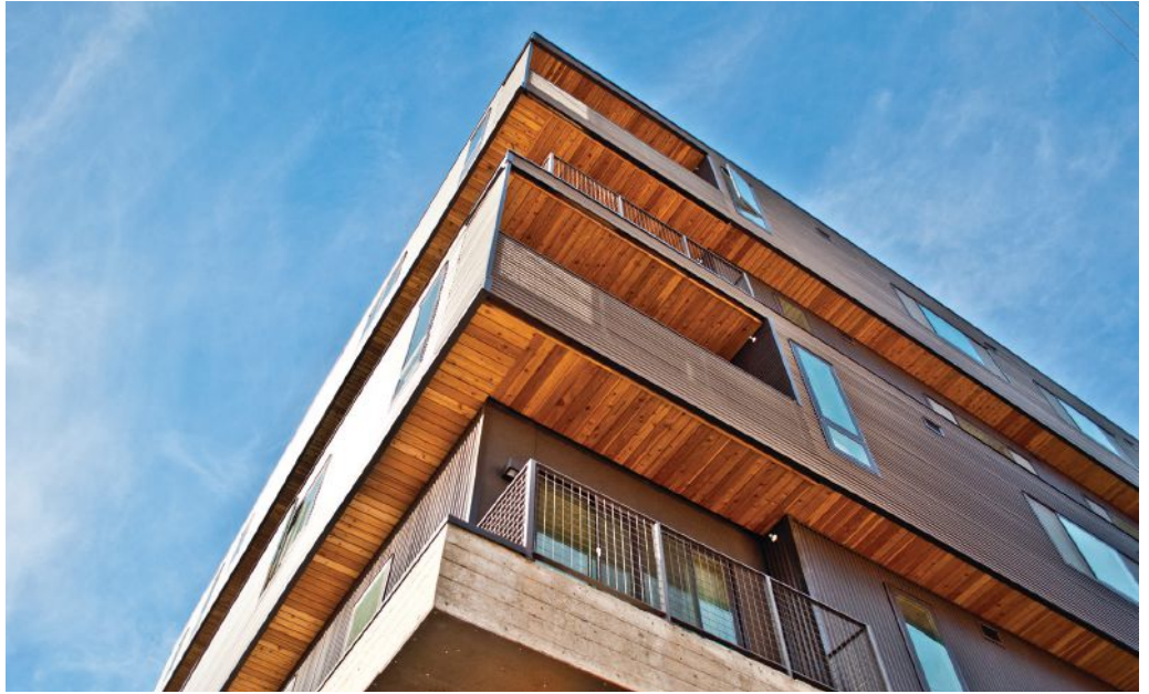
Warm cedar soffits are a natural counterpoint to the raw concrete base and industrial vibe of MOTO's metal panel cladding. Photo: Ronnie Leone
