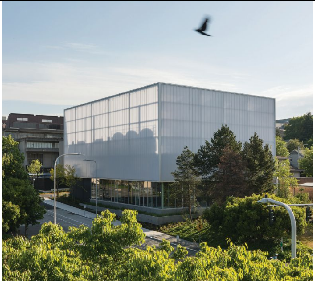
The Miller Hull Partnership's West Campus Utility Plant at the University of Washington proves that function can be a formal design expression.
