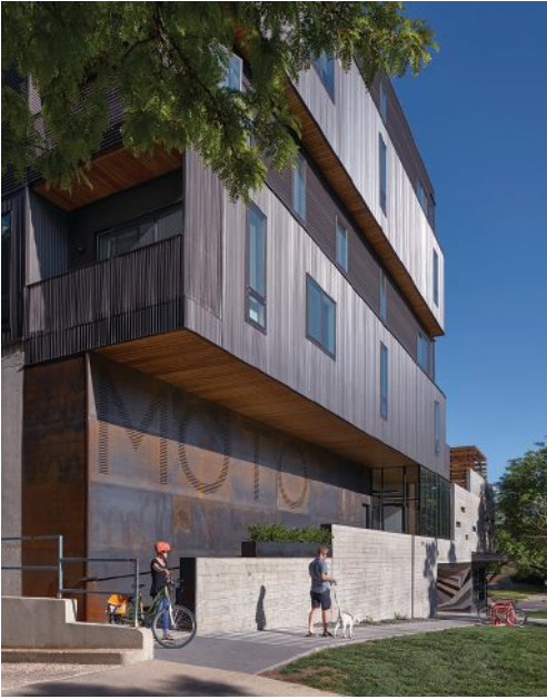
MOTO's cantilevered, stacked floors play with mass, creating a dynamic offset look that suits the fashionable neighborhood. Photo: Ryan Gobuty
