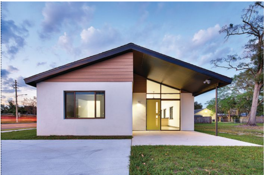
Each house is clad in stucco over concrete masonry unit walls, with an Azek deck-board rainscreen.
