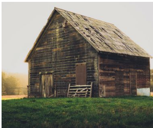
The gabled moderns of today are a contemporary take on the simple barn homes of the past and of vernacular architecture.
