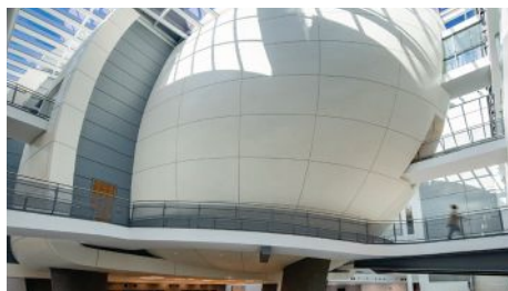
Steel Framing Duke Ellington School of the Arts Washington, D.C.
