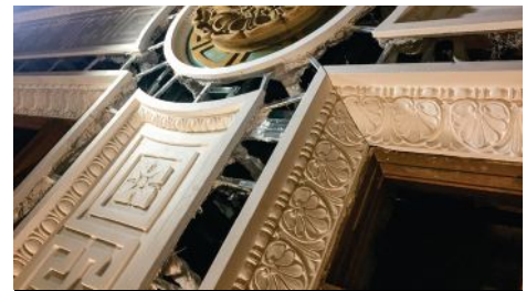
Interior Plaster 350 Bush Street San Francisco, California
