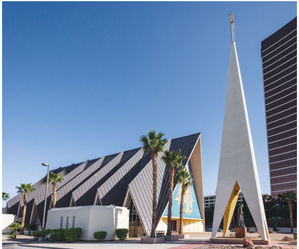
Guardian Angel Cathedral: Designed by pioneering African American architect Paul Revere Williams, the Guardian Angel Shrine opened in 1963 and became a cathedral upon the creation of the Diocese of Las Vegas in 1995. Its A-frame design features a large mosaic over the main entrance by Los Angeles artist Edith Piczek.
