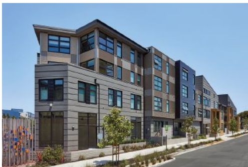
Located on the border of Emeryville and Oakland, this multifamily housing development on 3900 Adeline Street includes 91 residential and 10 work/live rental units.
