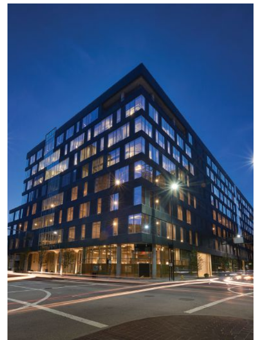
A high-performance building offers owners a greater return on investment than a conventional building due to reduced energy and operating costs, lower maintenance costs, improved functionality, and resilience after a catastrophic event.
