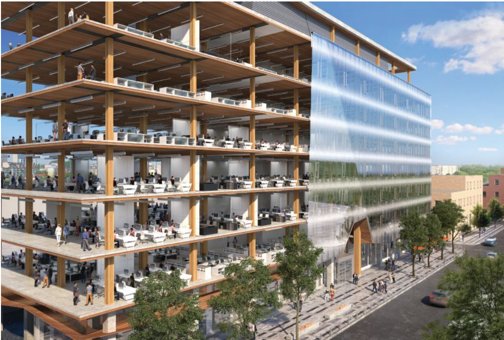
TOP LEFT A seven-story mass timber design has become integral to 77 Wade's marketing plan promoting its benefits to prospective tenants. TOP RIGHT Legacy on Park Avenue condo makes creative use of CLT in this curvaceous hybrid wood-frame mass timber design under construction. BOTTOM RIGHT A concrete podium wood-frame configuration offered significant value for money for architect Togawa Smith Martin's innovative double-podium design, supporting five levels of wood-framed structure and boosting density for the WREN Residences in Los Angeles.
