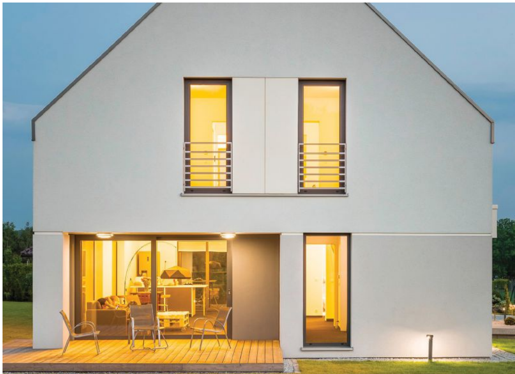
The Gabled Modern House as we commonly see it today—primarily in spec homes and custom builds.
