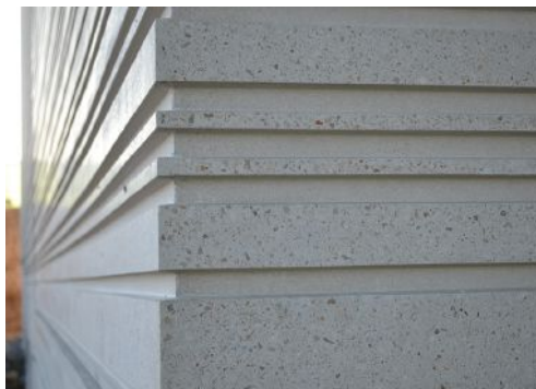
Precast concrete sandwich panels are cast in a flat orientation, so the front side is regularly the side that will be exposed to view in the final construction. This face can be made with virtually any type of finish.
