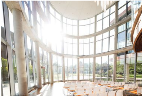
Uncontrolled glare and heat gain at Bowie State University could have made this space unusable.
