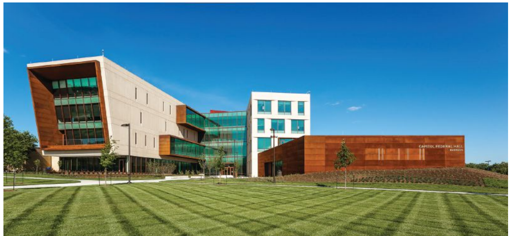
Precast was selected for ORNL research because of its high durability, best fit for commercial buildings, and certified quality control.
