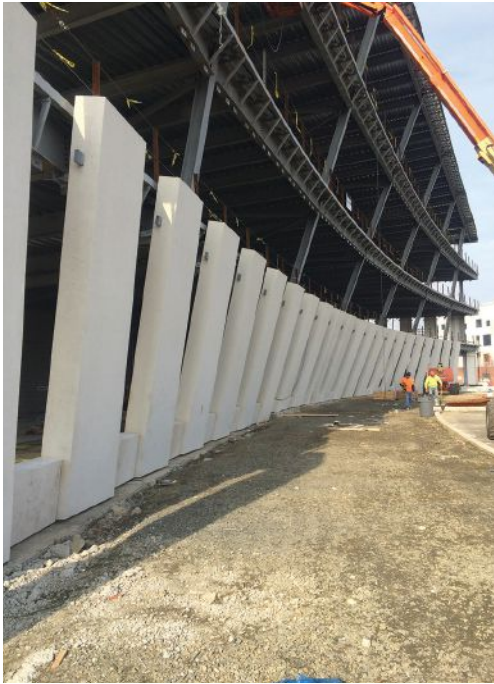
New thinner insulated wall panels will be lighter, easier to erect, have a broader range of uses, all with a higher R-value.
