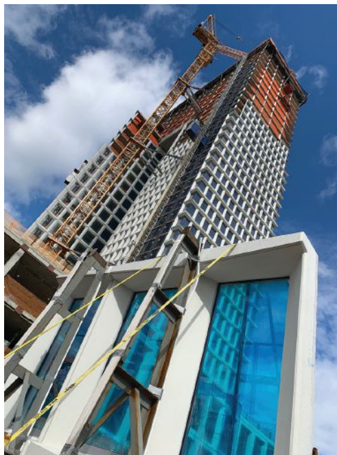
The repetitive nature of many fenestration patterns designed for building types such as hospitals, high-rise housing, and office buildings plays to precast concrete's strength in duplicating one pattern many times.
