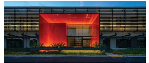
Lighting Design: Oculus Light Studio Architect: Shubin+Donaldson Architects Photos: ©Henri Khodaverdi
