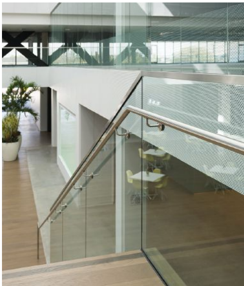
A correctly installed handrail system. Note that the brackets are not placed in between glass lites.
