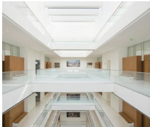
A glass railing system in a typical floor edge application. A cap rail is often used to maximize load performance.
