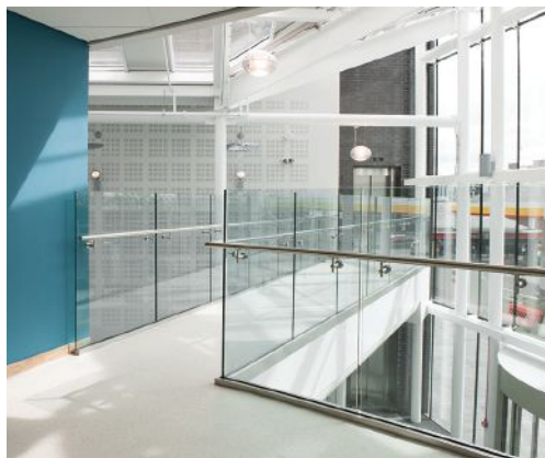
A glass railing system in a typical bridge application.
