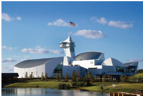
Discovery Center in the Discovery Park of America, Union City, TN Installing contractor: Ralph Jones Sheet Metal Inc. Architect: Verner Johnson Inc. General Contractor: Allen Searcy Builder-Contractor Inc. Photographer: hortonphotoinc.com Profiles: Lock-Seam, Snap-Seam Color: Silver
