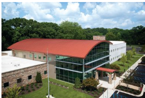
Jefferson County Western Health Center, Midfield, AL Installing contractor: CSC Roofing Architect: Birchfield Penuel & Associates General contractor: M.J. Harris Construction Services Owner: Jefferson County Department of Health Photographer: hortonphotoinc.com Profiles: Lock-Seam Curved Colors: Red
