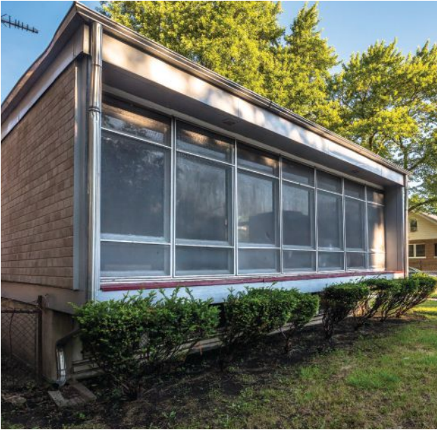
Above and Top Right: The Dr. E.J. Ingram House, designed in 1959 by the African American architect Roger Margerum
