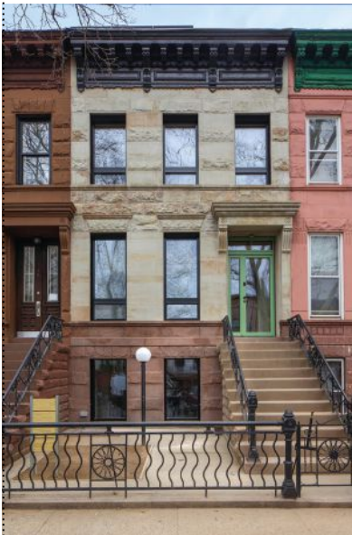
The front façade was fitted with retractable Hella shades that help prevent heat gain.
