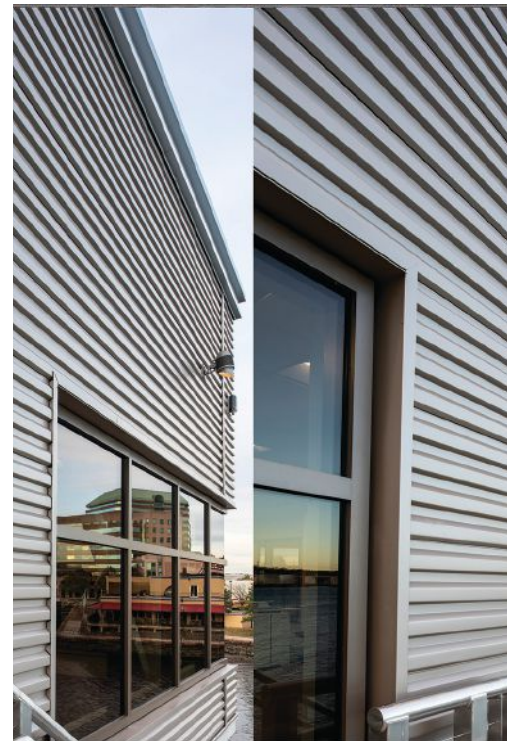
Canal Dock Boathouse, New Haven, CT
