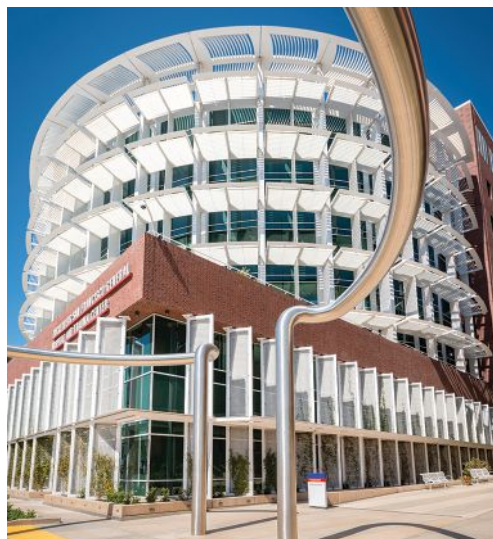
Zuckerburg San Francisco General Hospital Zuckerburg San Francisco General Hospital sits along the San Andreas Fault Line. Expansion joints were needed to connect the new hospital tower with the existing structure.
