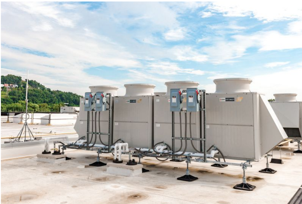
VRF's outdoor units are compact, quiet and lightweight.
