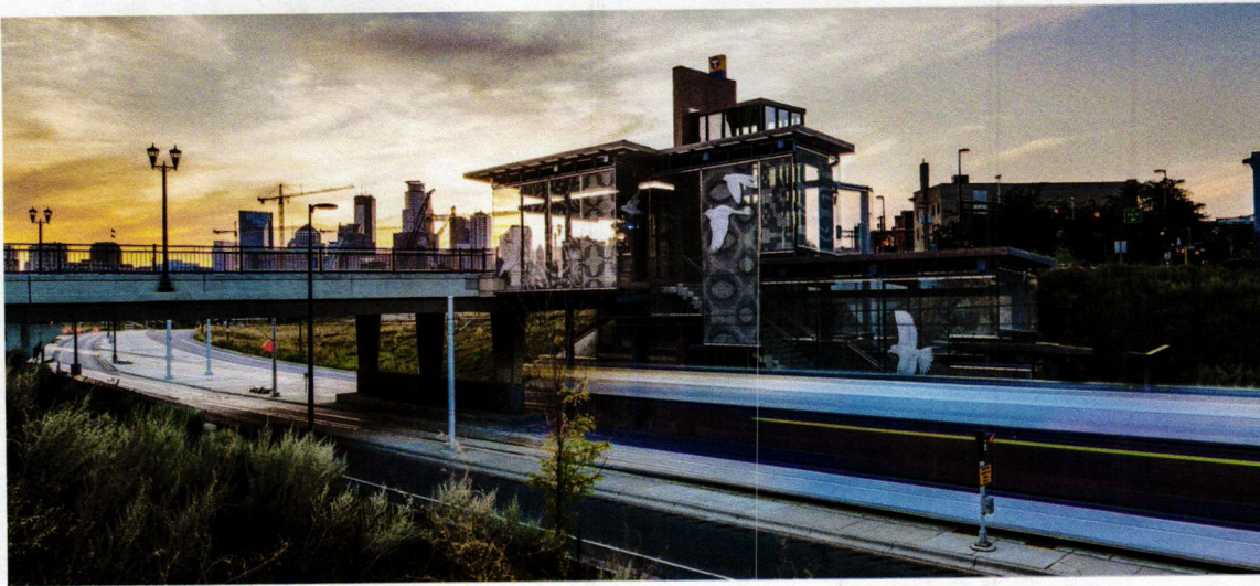
Left: 4RM+ULA collaborated with AECOM on the design and documentation of the 18 stations comprising the Twin Cities' Green Line Light Rail Transit.
