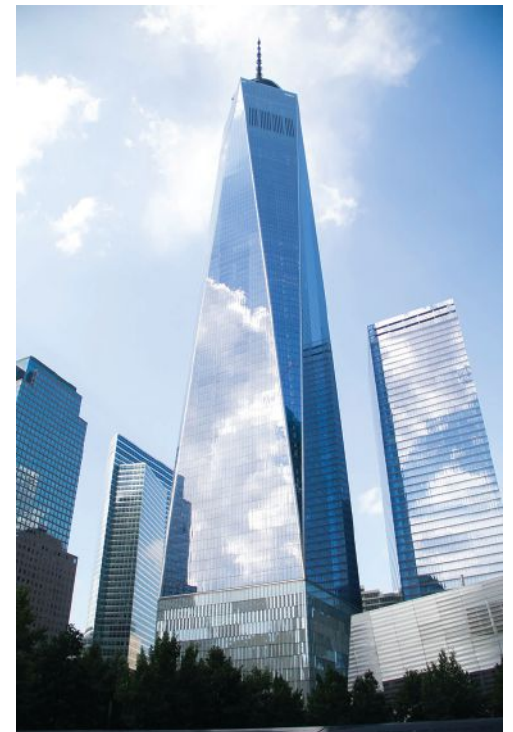
Figure 3. One World Trade Center, New York achieved LEED Gold Core and Shell certification using several advanced energy and water-saving technologies. In addition, the building used high strength “green concrete” produced using high volumes of fly ash. Photo: Spinel_S / iStock by Getty Images
