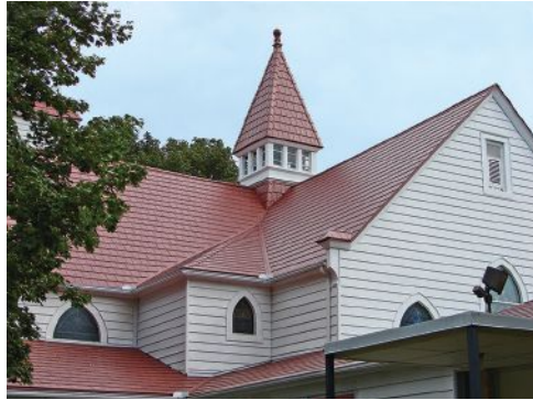
Slate roofing, wood shingle roofing, and wood siding have been popular for centuries and have been used to highlight various architectural styles throughout history. Now, steel roofing and siding is available that mimics these centuries-old products but with increased durability and performance.
