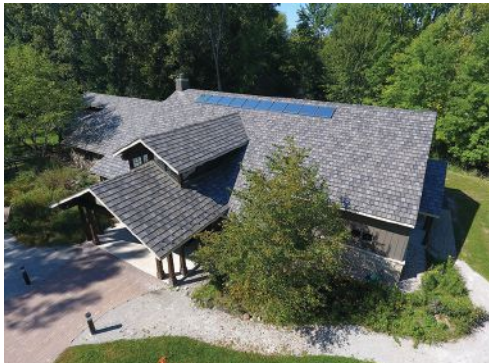
Steel roofing is available with a slate or shake look that mimics these centuries-old products but with increased durability and performance.
