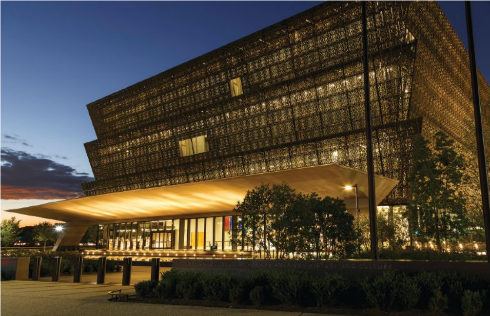
Figure 2. The Smithsonian National Museum of African American History and Culture, Washington, DC achieved LEED Gold certification by combining a wide range of operational and embodied impact reduction strategies including passive design strategies. Photo: Efrain Padro / Alamy Stock Photo.
