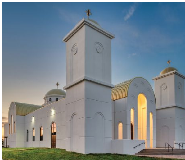
Photo: Courtesy of Tilt-Up Concrete Association. Photo by Michael Craft
