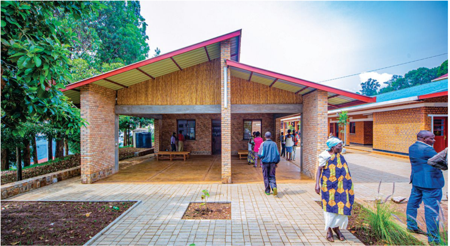
The buildings that compose the Masoro Health Center in Rwanda house curative services, administrative functions, preventative care, and maternity services.
