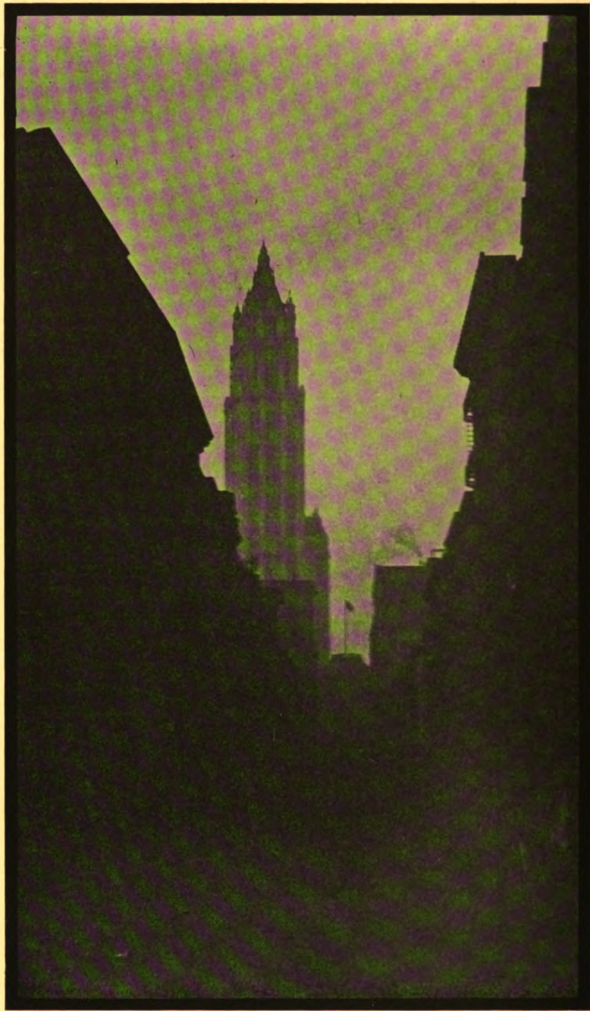
A CATHEDRAL VISTA (WOOLWORTH BUILDING, NEW YORK)
