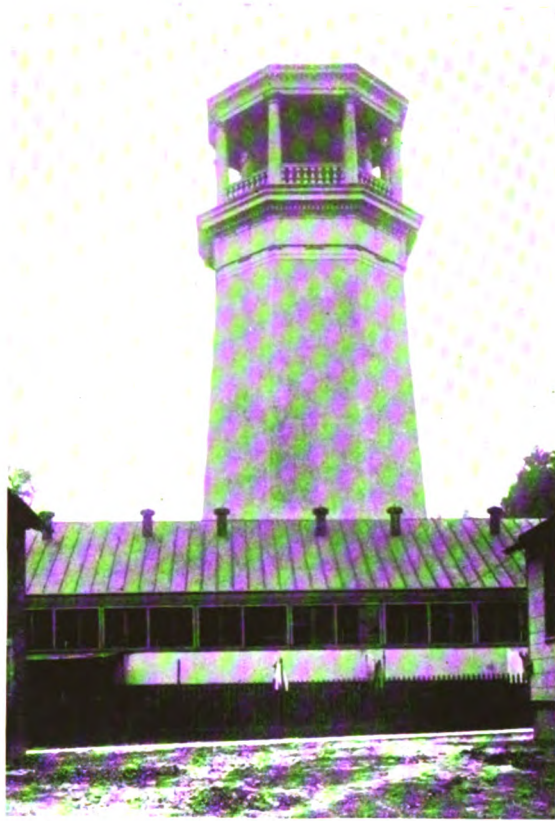
PHILADELPHIA.—Water-Tower on the Same Site. Approved by the Art Jury. The Improvement was Effected by Casing the Tower with Brick Covered with Stucco, and by Treating the Tank and Roof with Shingles.
