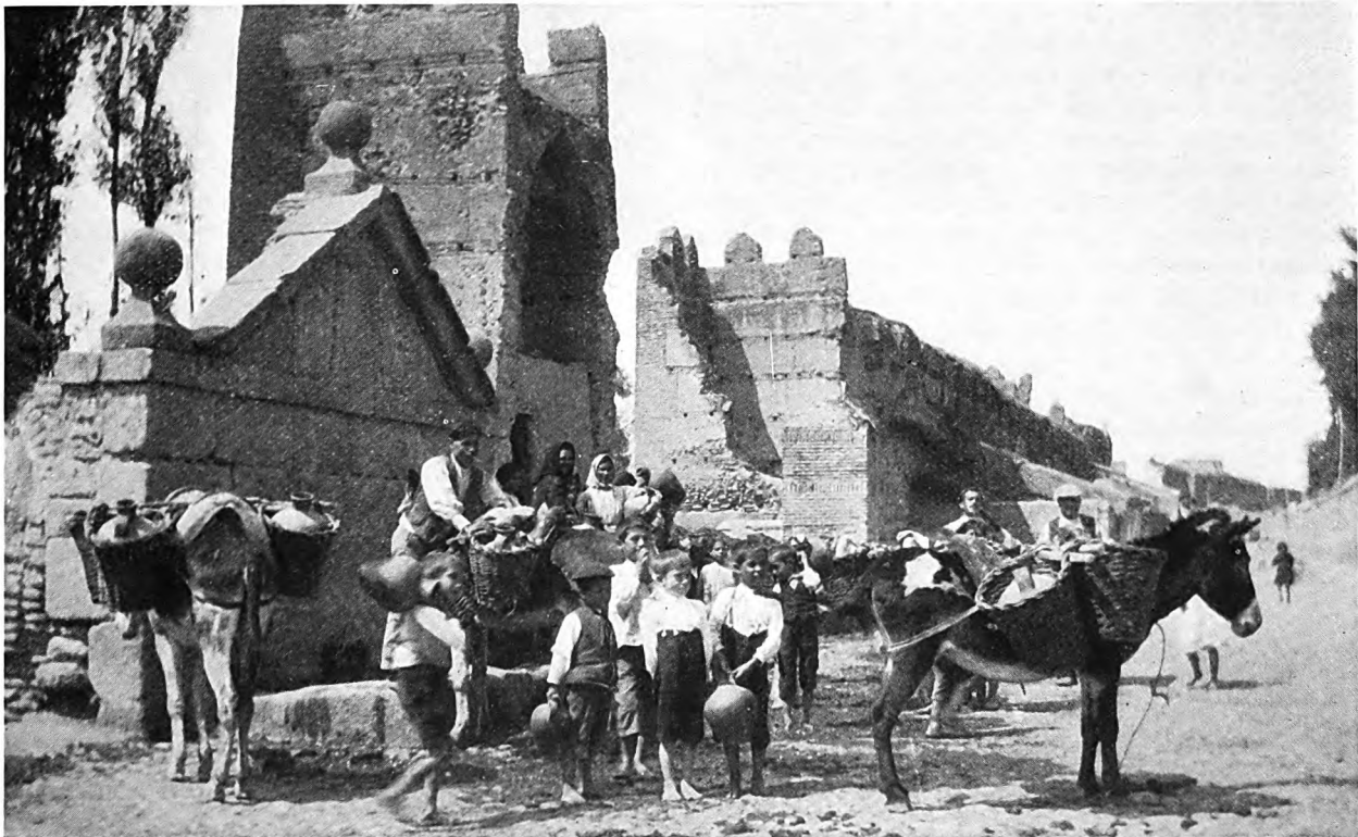
MADRIGAL DE LAS ALTAS TORRES—The Fountain by the Gate.
