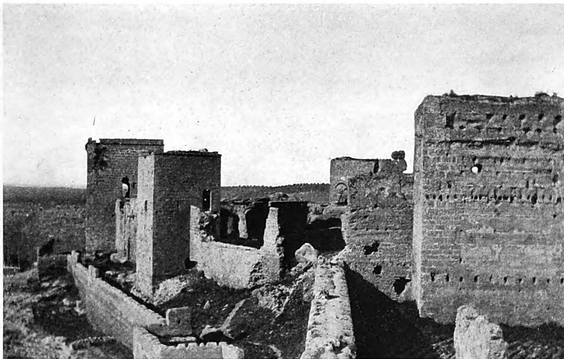
ALCALÁ DE GUADAIRA: CURTAIN-WALL AND BARBACAN
