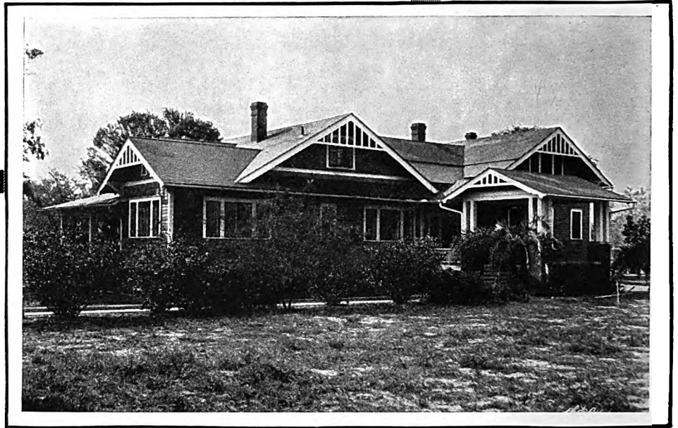
Home of Miss K. Jackson, Tampa, Fla.; Architect, F. J. Kennard, Tampa; Contractor, J. S. Sweet, Tampa
