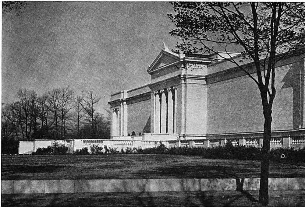
The Cleveland Art Museum, Cleveland, Ohio, Architects, HUBBELL & BENES
