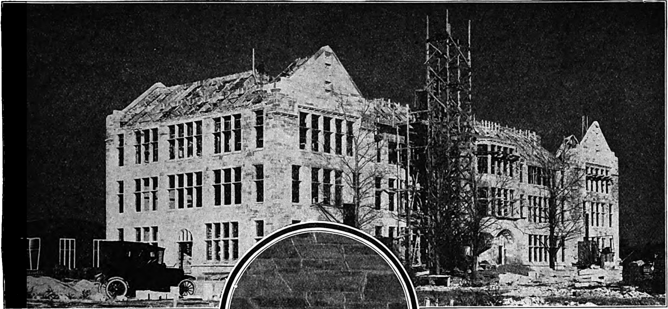
Evansville College Building, Evansville, Indiana. Messrs. Miller, Fullenwider & Dowling, Architects. In this construction, the masonry wall facing of Indiana Limestone has been most effectively combined with the cut stone trim.
