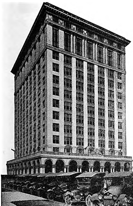
Texas Company Building, Houston, Texas. Original fixtures removed and Brascolites installed by the Brown-Woods Electrical Company of Houston.
