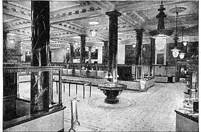
Remodeled fixture with one 300-watt Mazda lamp and three 40-watt bulbs—420 watts—four foot-candles.
