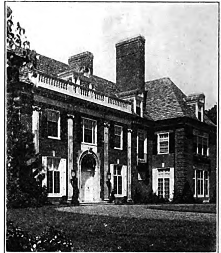
Residence of Mrs. Leland H. Ross at Madison, N. J. Behr & Smith, Associate Architects
