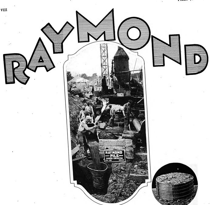
For twenty-three years the Raymond Pile has demonstrated that certainty of construction and increased carrying power are attained by placing the concrete in a spirally reinforced shell, which shell remains permanently in the ground.
