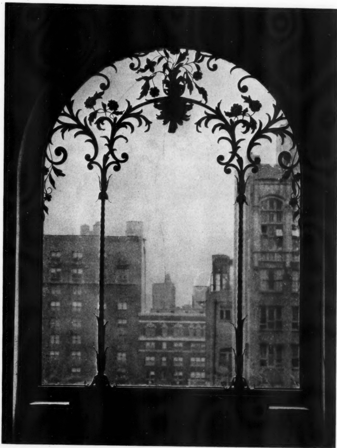
WINDOW GRILLE OF WROUGHT IRON WITH HAMMERED LEAVES APPLIED TO THE IRON STRUCTURE
