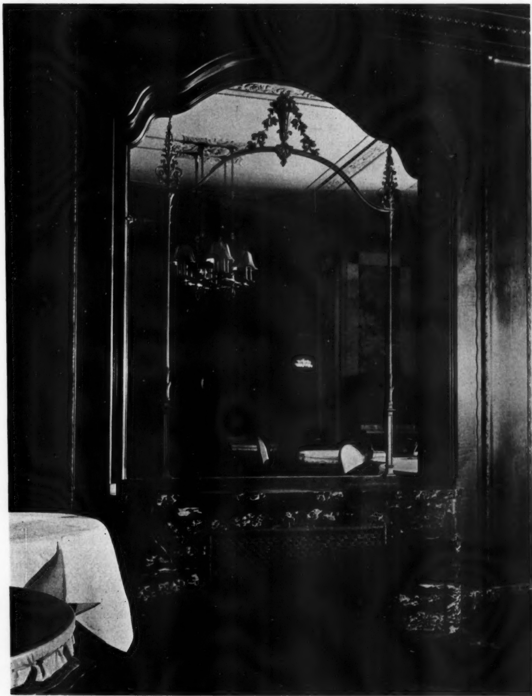
GRILLE AND MIRROR FRAME OF CAST BRASS NICELY CHASED USED TO GIVE INTEREST TO THE PLAIN MIRROR SURFACE
