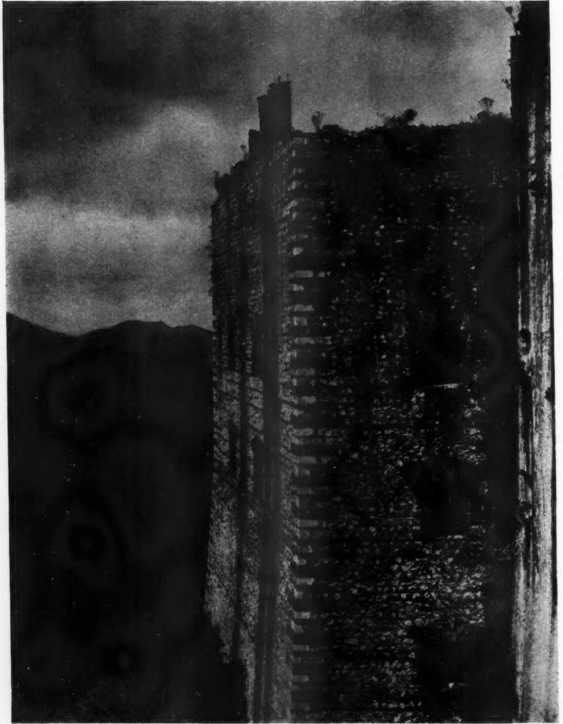
A FIELD OF RANDOM MASONRY BORDERED BY BRICK AND CUT-STONE QUOINS IN THE CITADEL OF LA FERRIERE, HAITI
