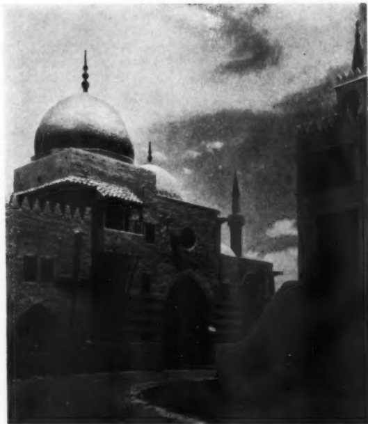
AN EXPERIMENT IN ADAPTING ARCHITECTURAL STYLE TO LANDSCAPE MUNICIPAL BUILDING, OPA-LOCKA, FLORIDA
