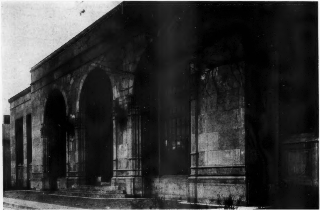
ST. LOUIS PUBLIC LIBRARY. WILBUR T. TRUEBLOOD & HUGO K. GRAF, THE ARCHITECTS GEORGE O. CARPENTER BRANCH, GRAND BOULEVARD AND UTAH PLACE
