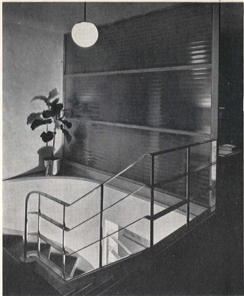
STAIRWAY DETAIL, RESIDENCE OF MR. AND MRS. E. P. MATHER MINNEAPOLIS, MINN.
